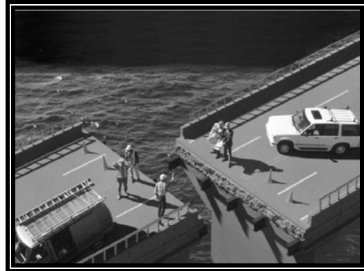
Consequences of using inconsistent coordinate systems (photo courtesy of Zurich North America Inc.).
