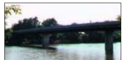
Pont de Chiefswood
