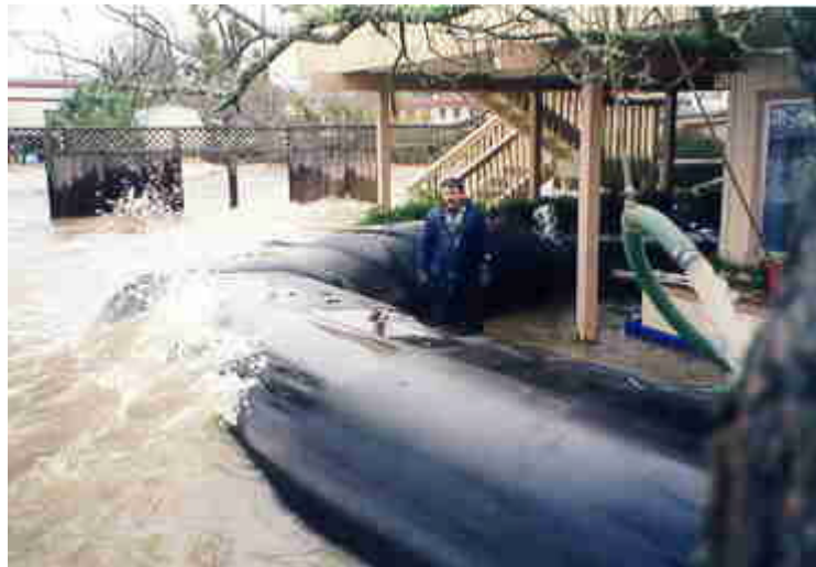
FIGURE 4.4.9 TUBULAR WATER-FILLED SYSTEMS: EXAMPLES OF APPLICATION “WATER STRUCTURES”
