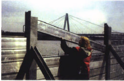
FIGURE 4.3.4 GOH DPS 2000 SYSTEM: INSTALLATION
