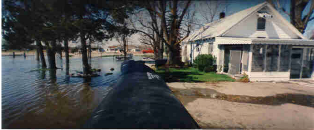
FIGURE 4.4.3 TUBULAR WATER-FILLED STRUCTURES: PORTABLE DAMS (“WATER STRUCTURES”)
