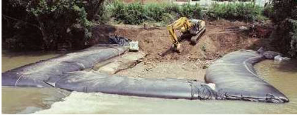
FIGURE 4.4.6 TUBULAR WATER-FILLED STRUCTURES: FLEXIBILITY, CORNERS, TUBE COUPLING (“AQUA BARRIER”)
