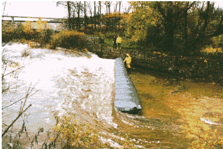
FIGURE 4.4.1 WATER WALL SYSTEM
