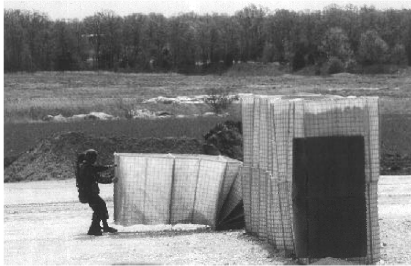
FIGURE 4.1.3 HESCO CONCERTAINER INSTALLATION: STRETCHING THE CAGE
