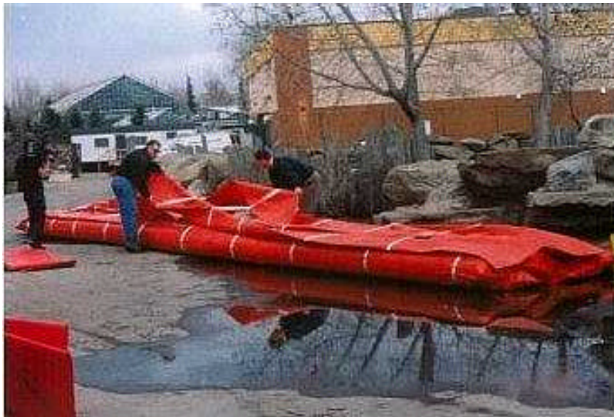
FIGURE 4.4.7 TUBULAR WATER-FILLED STRUCTURES: “CLEMENT” SYSTEM INSTALLATION
