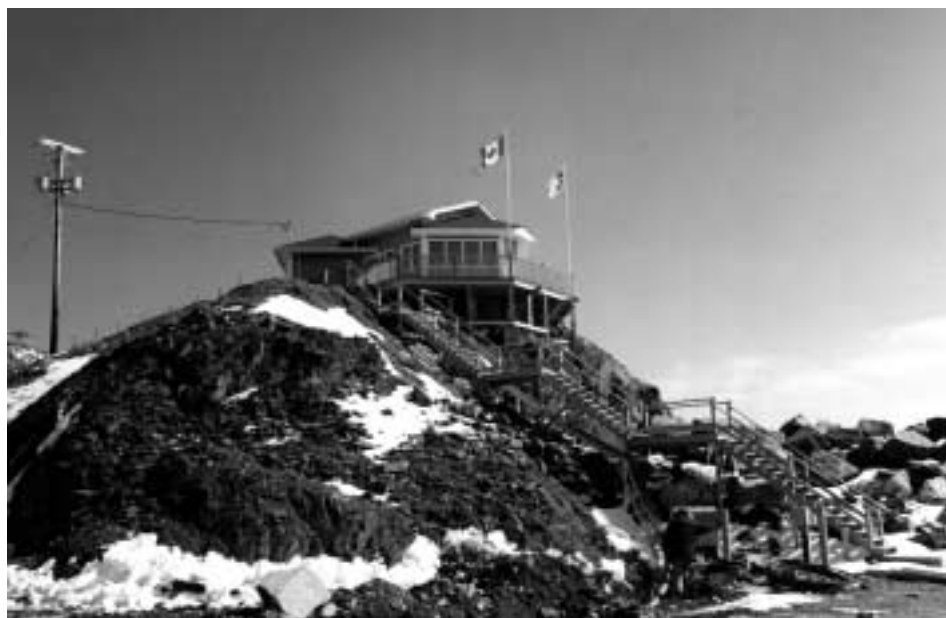
The new Morgan & Hawe Memorial Building is home to the Harbour Authority of Port de Grave.
