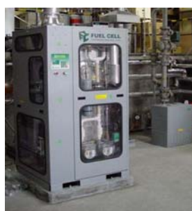
Figure 16: Stationary 5 kW (courtesy of Fuel Cell Technologies)
