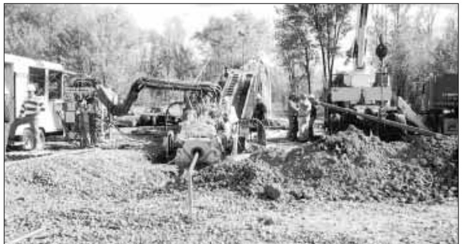
Figure 10. A directional drilled crossing
