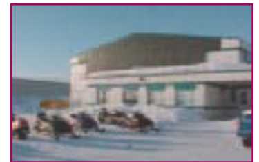
Alaittuq High School Solarwall
