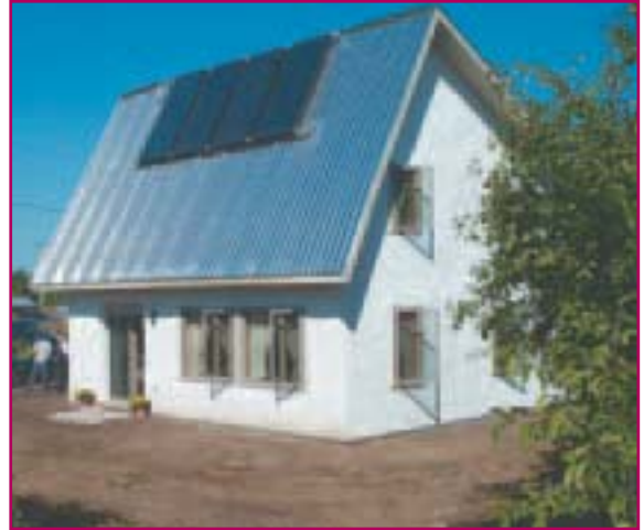
The Kanata Healthy House with solar panels installed
