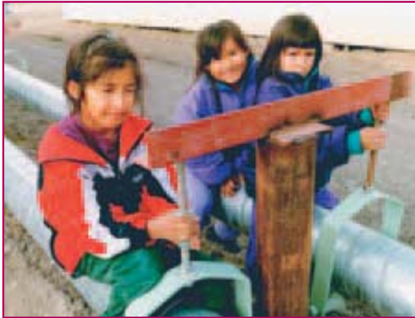
Above ground piping
