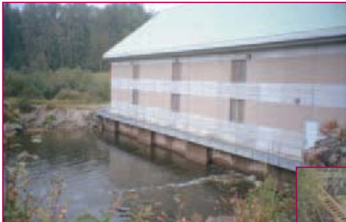
Black River Hydro Station
