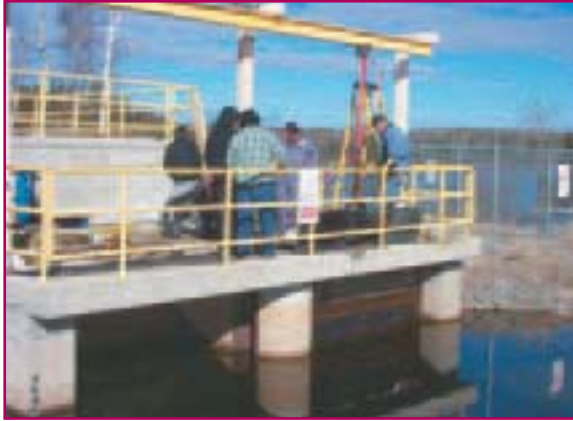
The Hydro Station undergoing repair and maintenance
