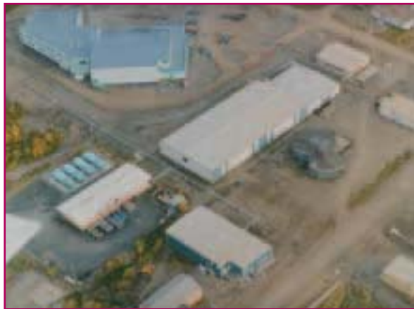
Aerial view of buildings serviced by district heating system
