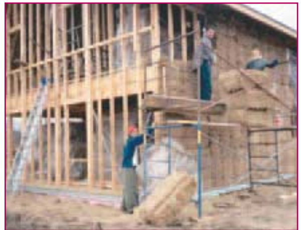
Kanata Healthy House Under Construction
