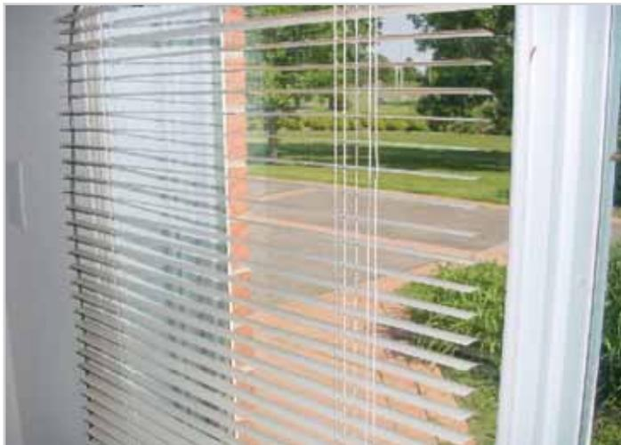
**Figure 2** Benchmark shading configuration – Venetian blinds in the down position with slats horizontal
