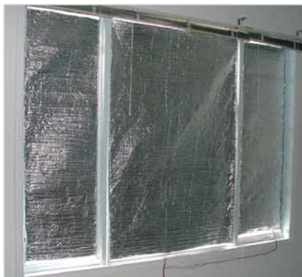
Figure 1 Three reflective shades mounted on the interior of a south-facing window
