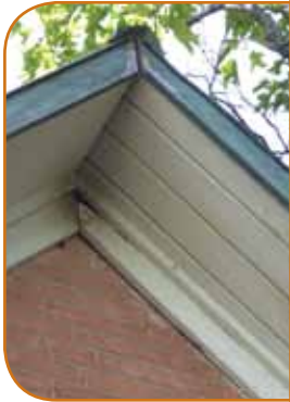
Look for gaps in trim for bat entry sites.
