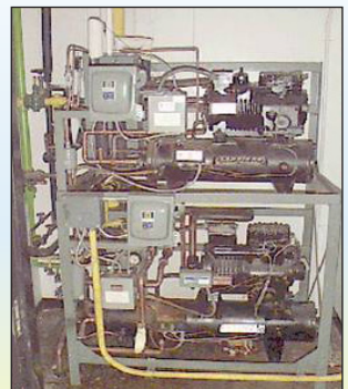
Walk-in refrigerator compressors
