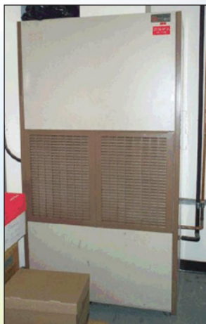
Air conditioning evaporator
