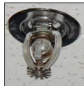
Showerhead of fire extinguishing system
