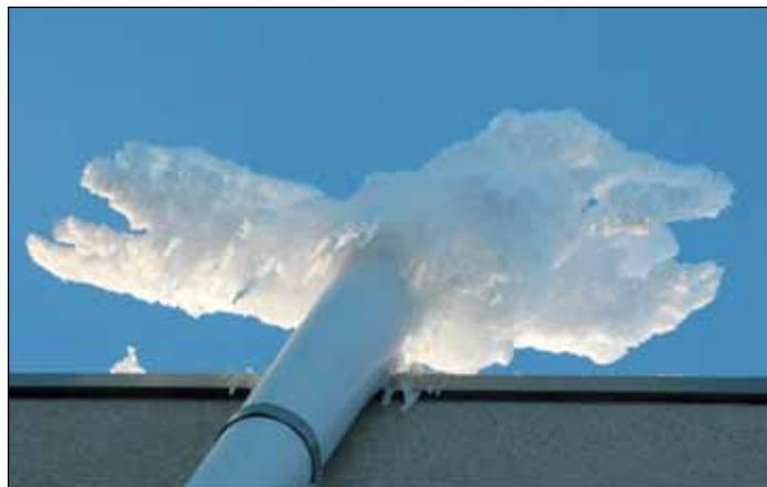
**Figure 1** Frost covered radon vent in Winnipeg
