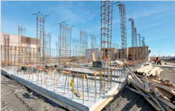
Nitrate preservation facility construction, November 13, 2009 Photographer: Gordon King
