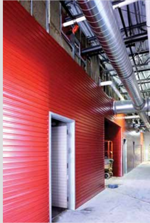
Inside the nitrate preservation facility, March 2, 2010 Photographer: Gordon King
