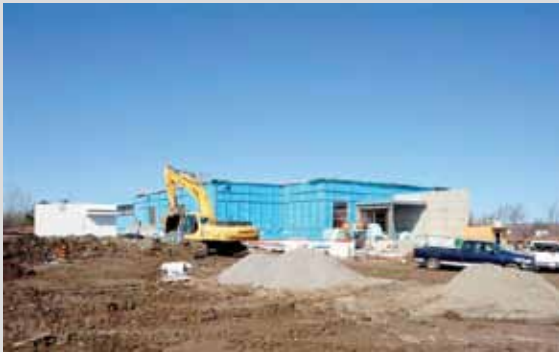
Construction of nitrate preservation facility, March 21, 2010 Photographer: Gordon King
