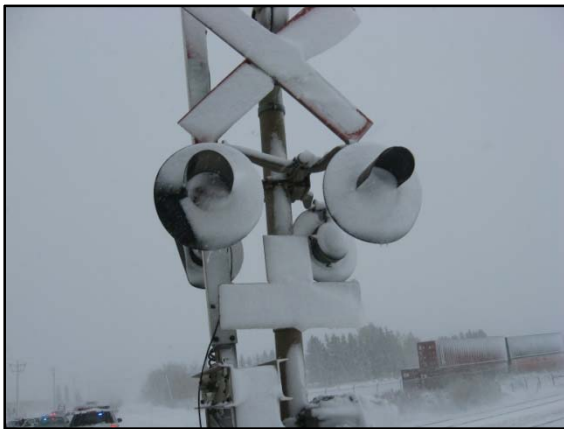
Photo 1. North signal, northward-facing lights
