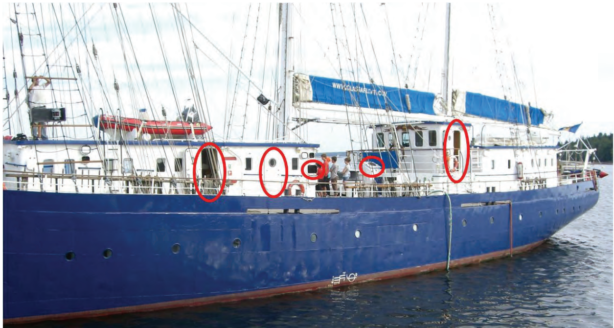
Photo 3. Some critical port side openings
