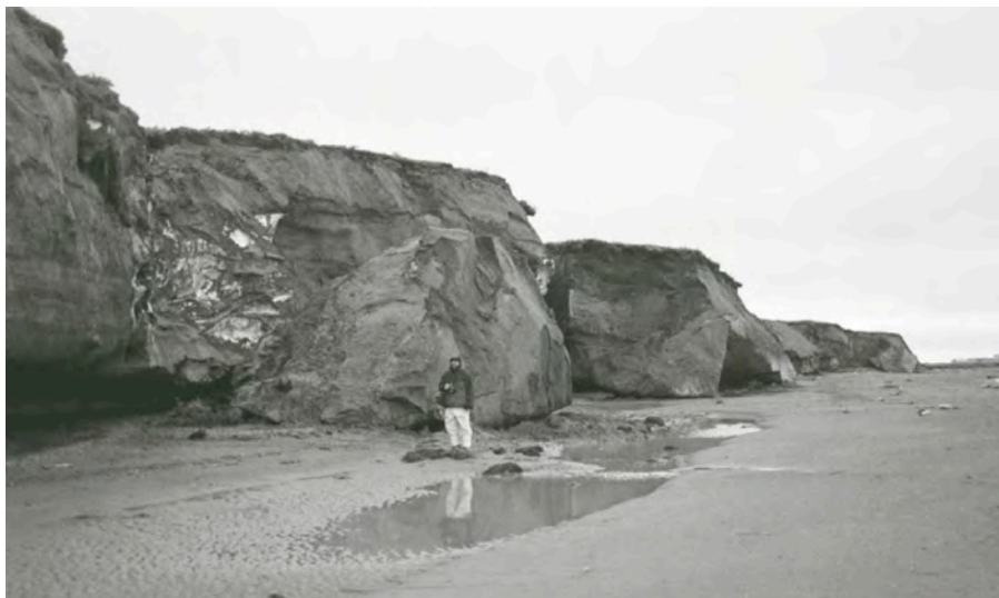
Figure 6 Photographs show, at the base of the bluff, an example of morphodynamic change in a thermo-erosion notch composed of frozen fine sand and silt with scattered cobbles and boulders: (a) development of the niche, and (b) later block failure of the same cliff.
