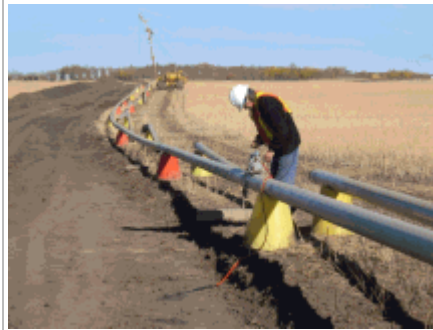
Image #6: NDT pipeline inspection, using industrial radiography equipment
