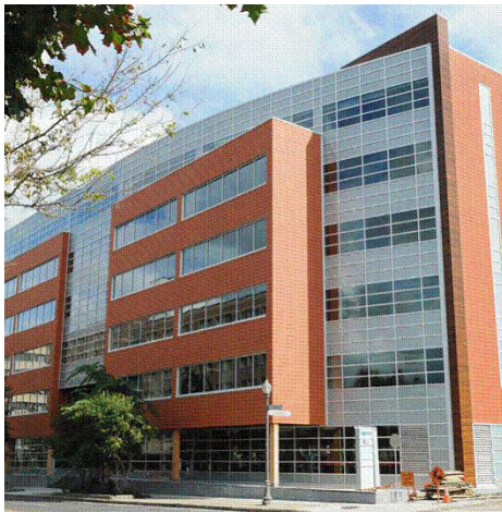
A 6-storey glulam post-and-beam structure with reinforced concrete cores in Quebec City, Quebec. Photo Credit: CSN-FONDACTION/ Nordic Engineered Wood
