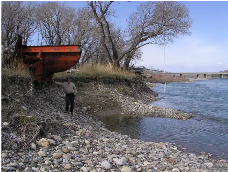
Figure 14. South bank of the Oldman River immediately east of the Highway 2 bridge (in background), west of Fort MacLeod (facing west). Note massive snow plow scoop wedged into the bank. The spring and seep habitat required by S. bertae is so small that such anthropogenic disturbances could completely destroy the habitat. (Photo courtesy of Jennie Knopp.)
