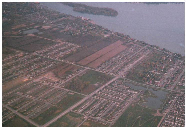
Figure 8. Stormwater ponds, Windsor, Ontario Photo by: D.W. Alley, 2007
