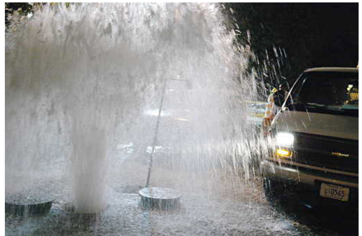
Figure 1. Geyser resulting from a water main break Source: http://www.flowmetrix.ca/Leak.php
