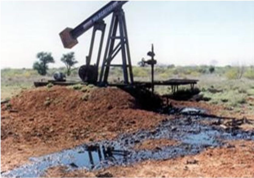
Figure 6: Leaking oil well Source: Texas Land and Mineral Owners Association, 2005
