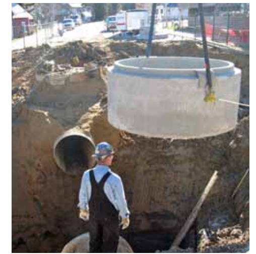
Installation of oil-grit separator
