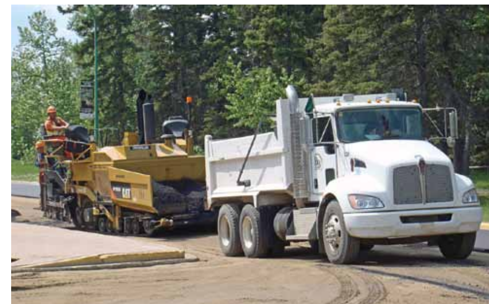
Finishing paving above the oil-grit separator
