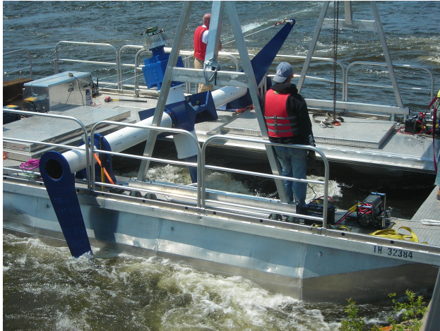
Figure 5 New Energy Corporation: Deployment of 25kW EnCurrent Power Generation System
