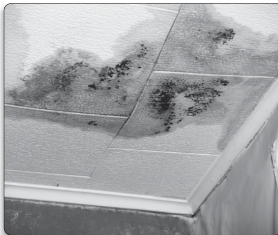
Mold can grow on wet ceiling tiles
