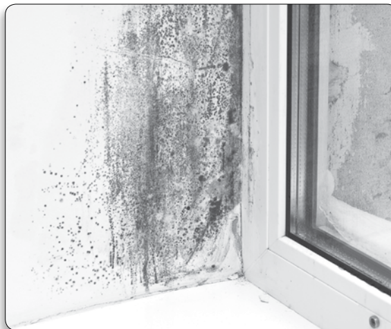
Mold can grow on damp drywall
