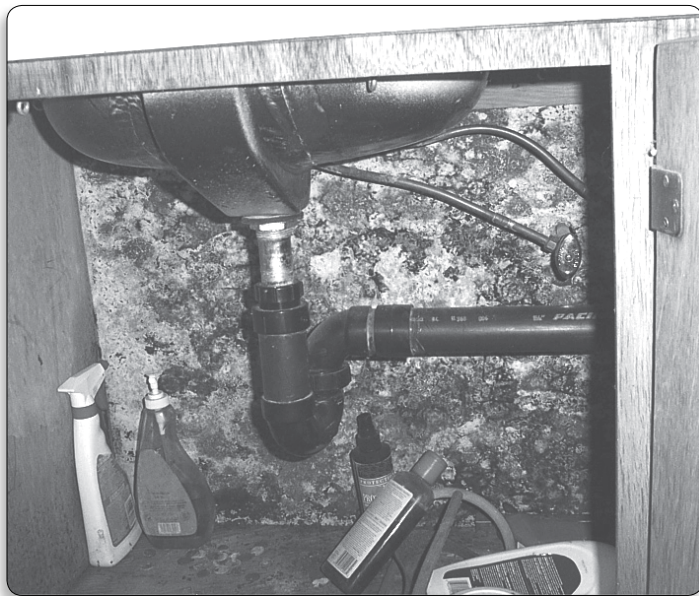
Plumbing leaks can lead to mold
