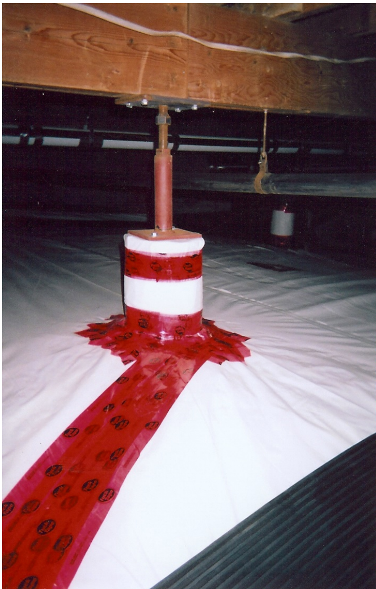
Photo 10: Mold from the floor joists has been physically removed by grinding, sanding and scraping followed by washing and HEPA vacuuming. Piping and pipe insulation have been repaired and properly sealed.
