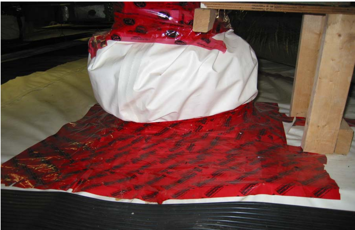
Photo 8: Tape is in good condition and has not detached from the floor barrier. The Permalon™ wrapping around the concrete piles is in excellent condition. Although crude looking, the wrapping of the piles provided a durable and well sealed system to isolate the piles.
