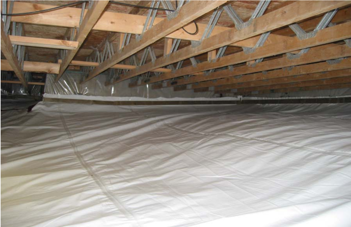
Photo 5: Floor barrier is clean and in excellent physical condition. The Permalon™ floor barrier extends part way up the exterior crawl space wall and merges with poly sheeting, which covers the remaining exterior walls. Wooden joists show no signs of mold re-growth or deterioration from extensive bleaching methods.
