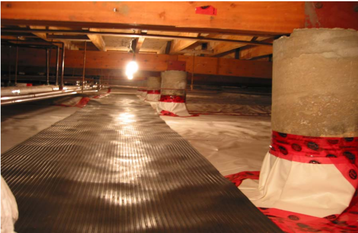
Photo 9: Floor barrier, tape and rubber mats are in excellent condition. Floor barrier extends up the concrete piles and is sealed to enclose the base of each column.
