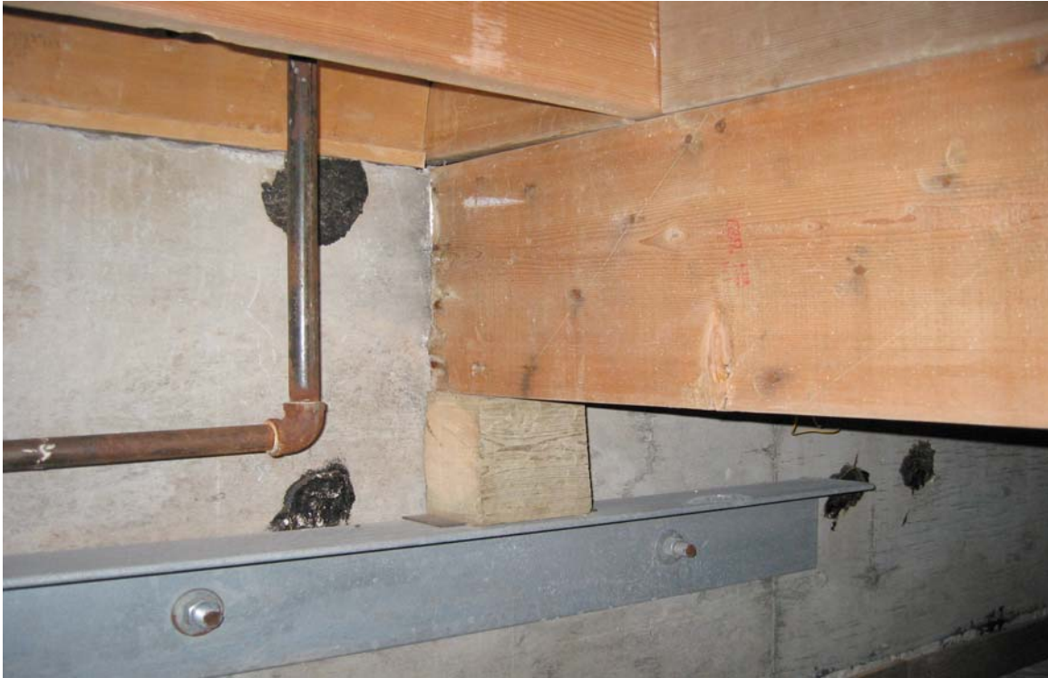
Photo 6: Additional structural supports are in good condition and functioning properly.
