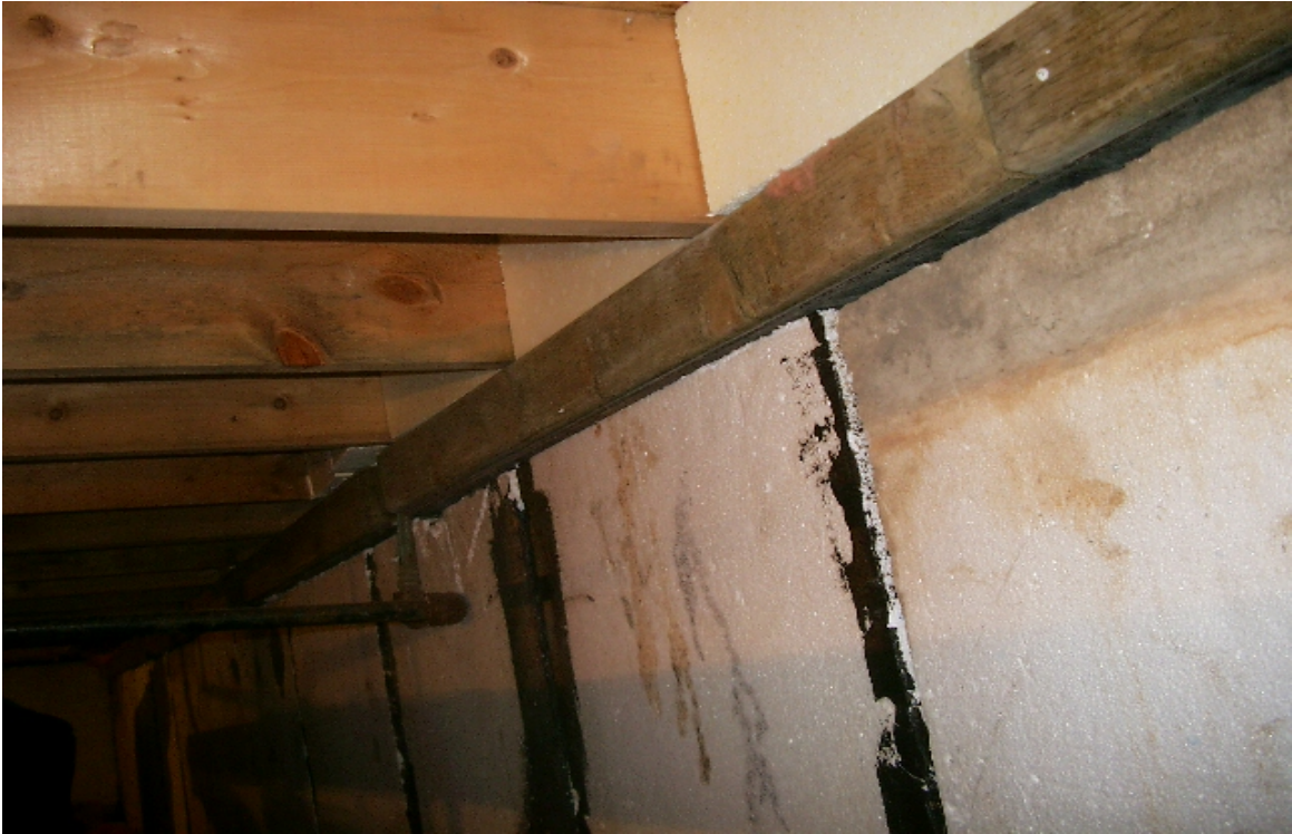
Photo 4: Exterior walls were insulated from the interior side of the crawl space.
