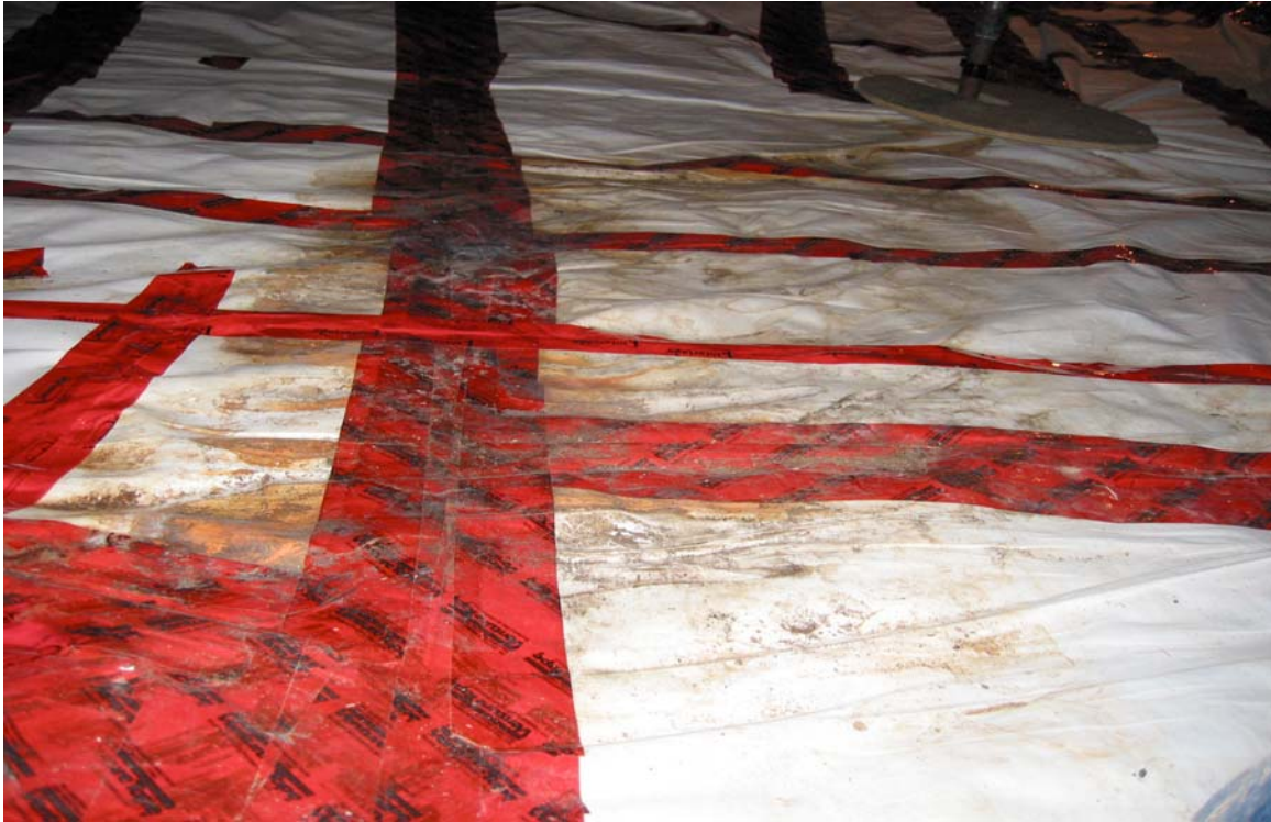
Photo 4: Crawl space floor is dirty and shows evidence of water entry from the main floor.
