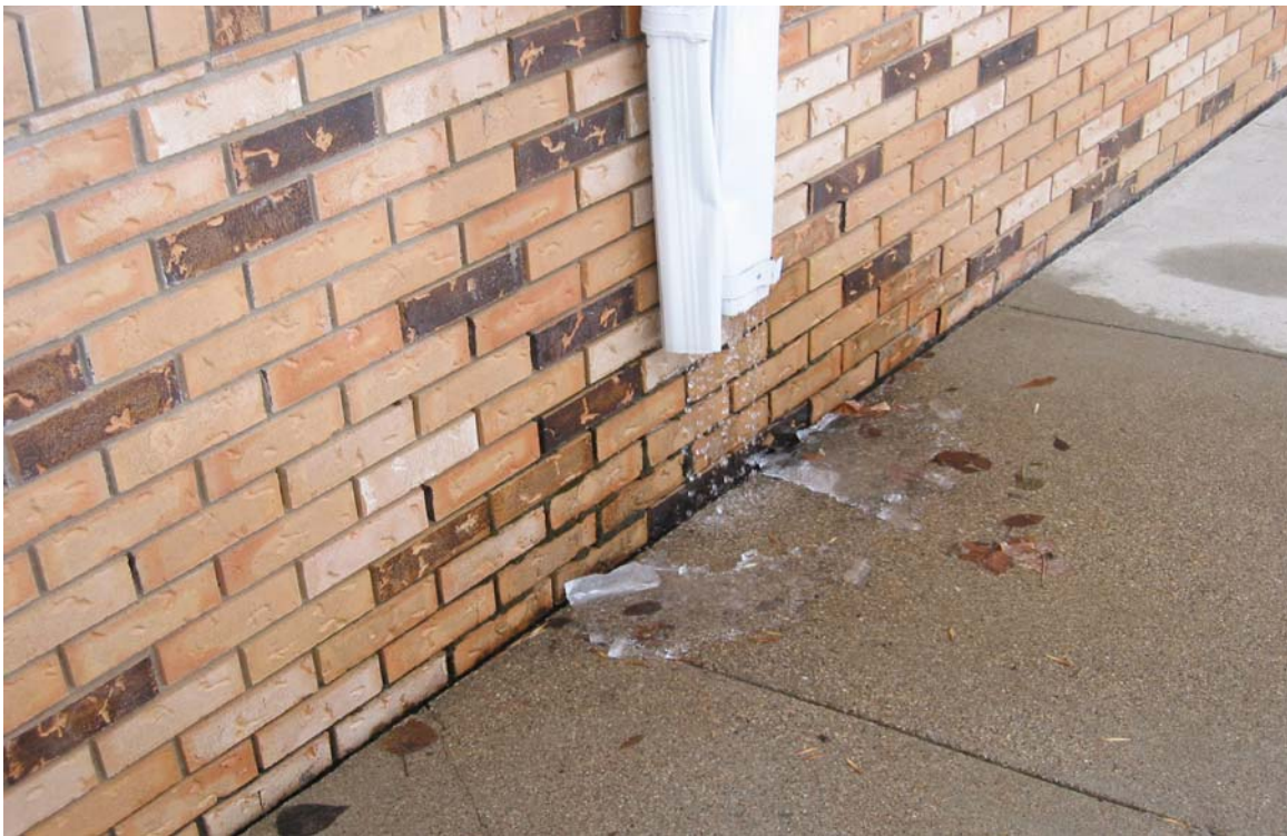
Photo 7: Some downspout extensions are missing and water is not moved away from the exterior walls of the crawl space.
