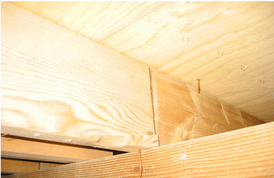
Photo 5: Floor joists and plywood subfloor are in good condition and show no signs of mold re-growth.
