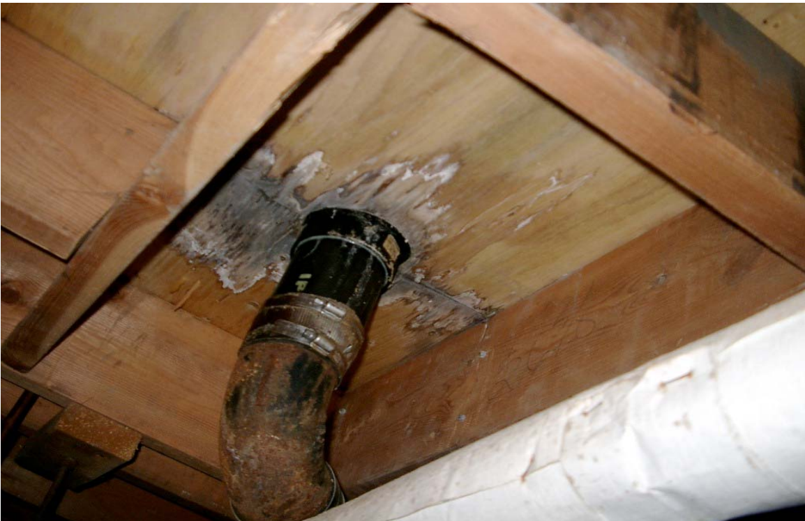
Photo 1: Visible mold and discoloration on the subflooring and floor joists.
