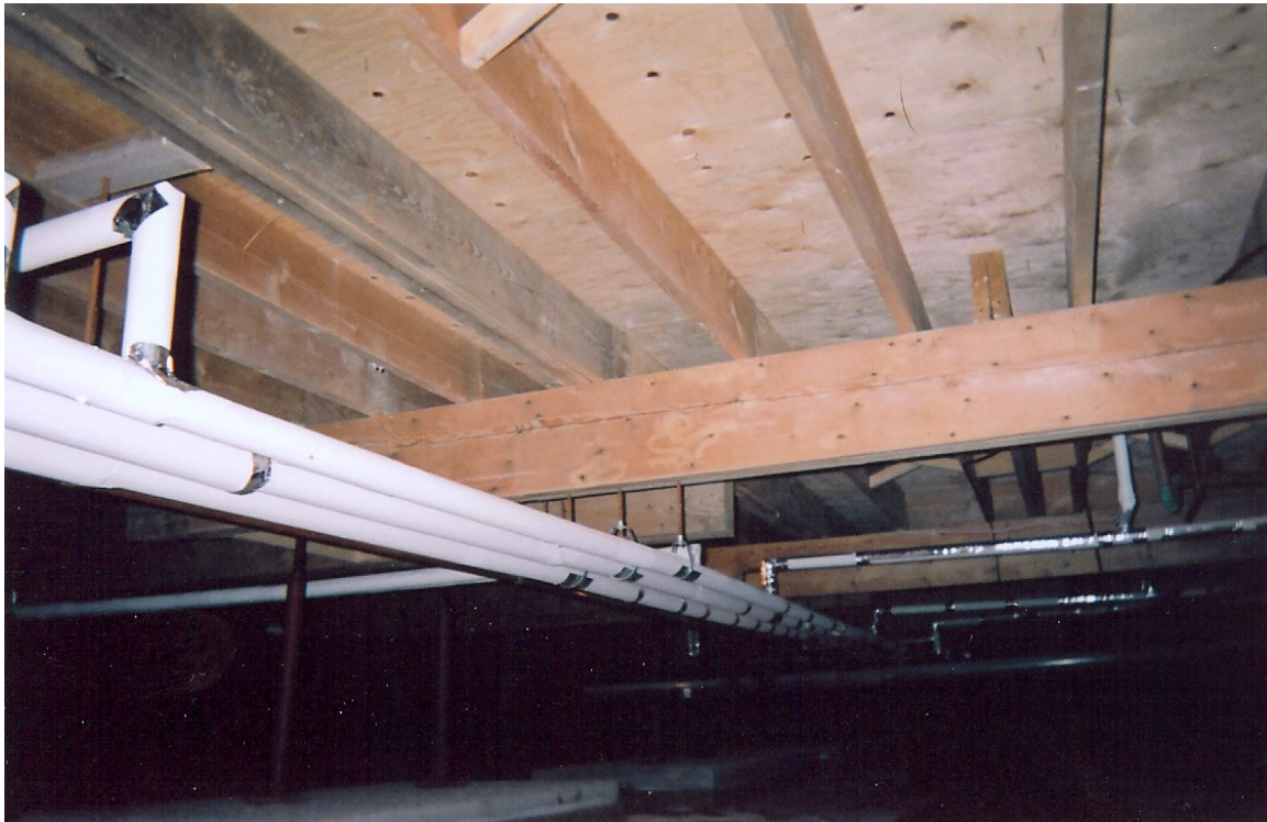
Photo 10: Mold from the floor joists has been physically removed by grinding, sanding and scraping followed by washing and HEPA vacuuming. Piping and pipe insulation have been repaired and properly sealed.
