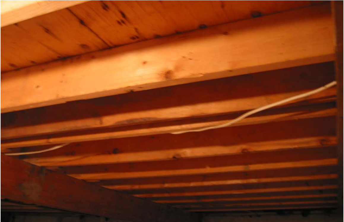
Photo 10: Plywood subfloor and floor joists are in good condition and show no evidence of mold re-growth.
