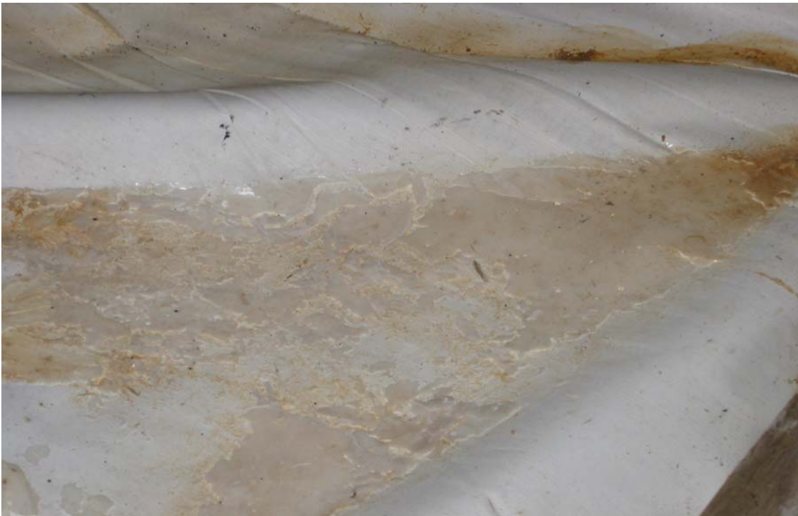
Photo 4: White crystals (either bleach residue or mineral deposits) are found on the floor barrier.
