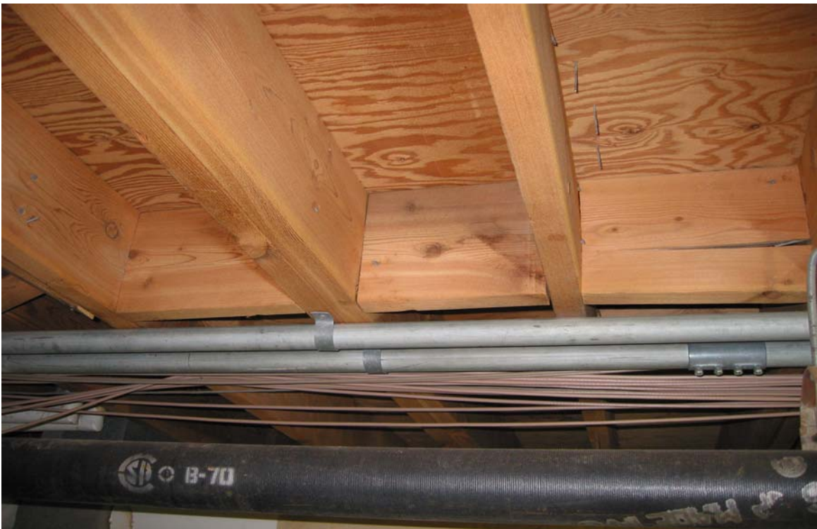
Photo 6: Floor joists and sub-flooring are in excellent condition after sand-blasting.
