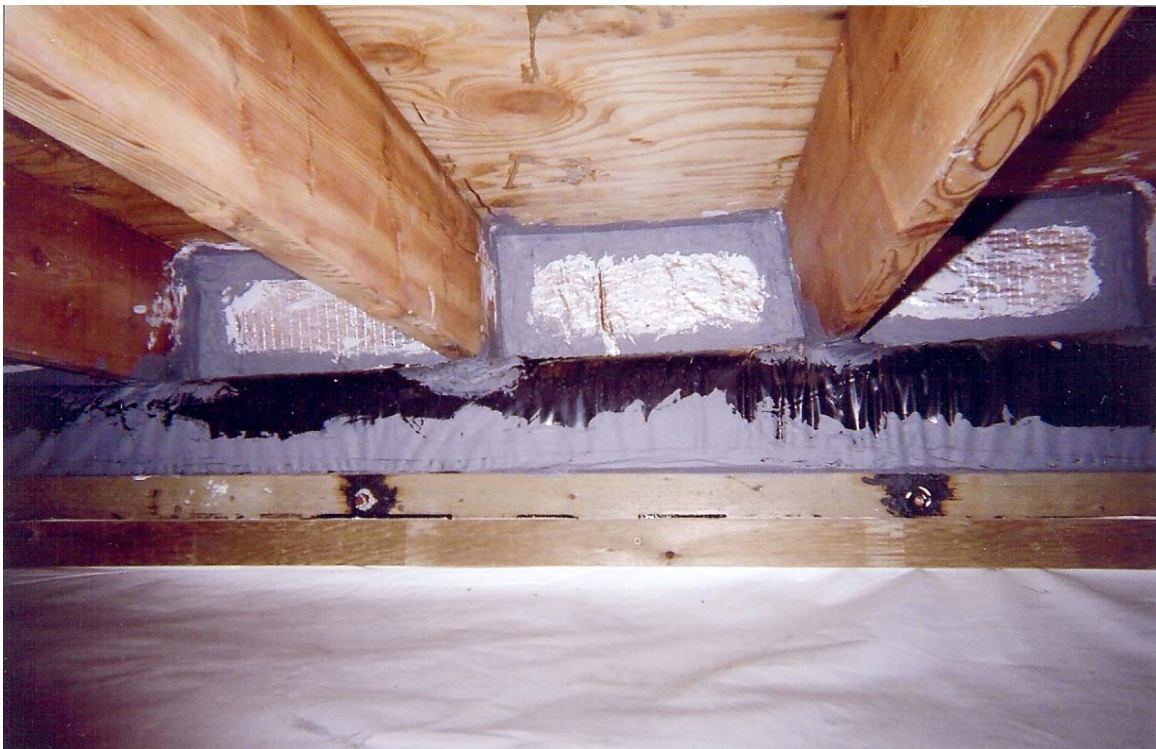
Photo 7: Foil faced insulation installed on the exterior rim joists. The plywood subfloor and the floor joists show no signs of mold re-growth or deterioration. Floor barrier is well attached and sealed to the existing glass fibre insulation system at the exterior wall.
