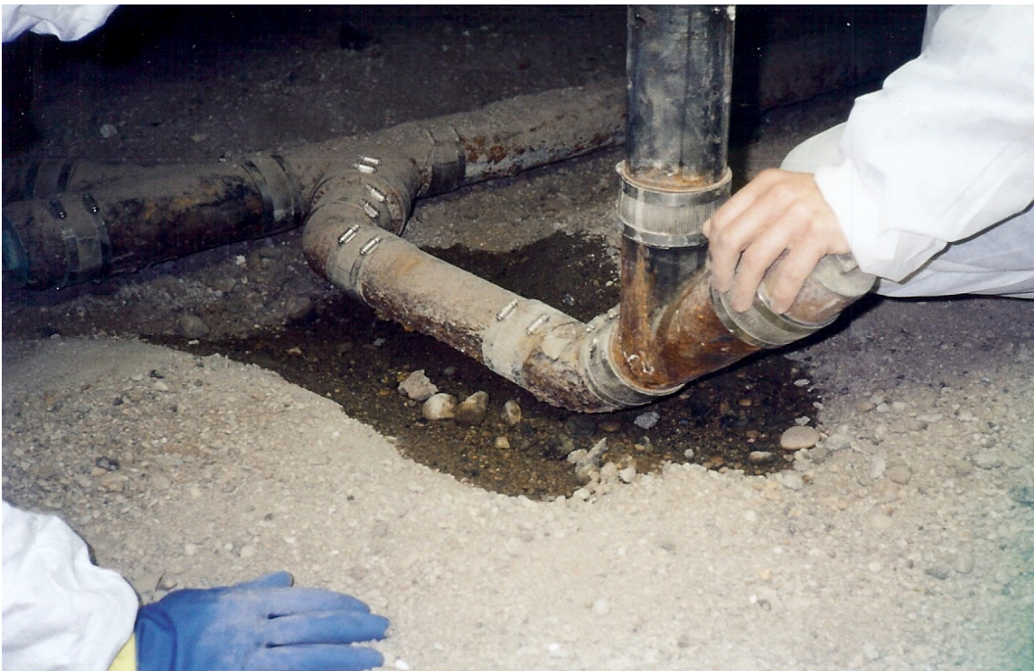
Photo 4: Old, corroded piping was a source of water entry into the crawl space.
