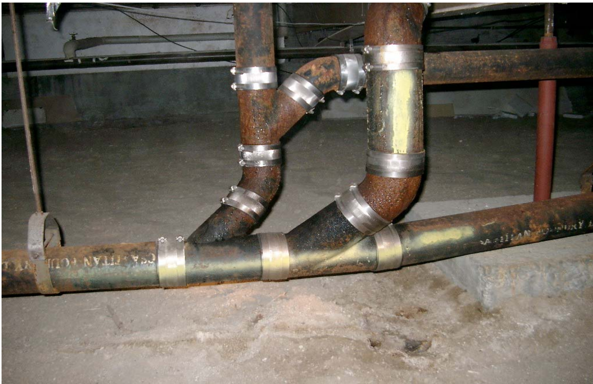
Photo 3: Piping/plumbing within the crawl space area showed signs of extensive rusting and deterioration. Perimeter insulation was poorly installed or missing.
