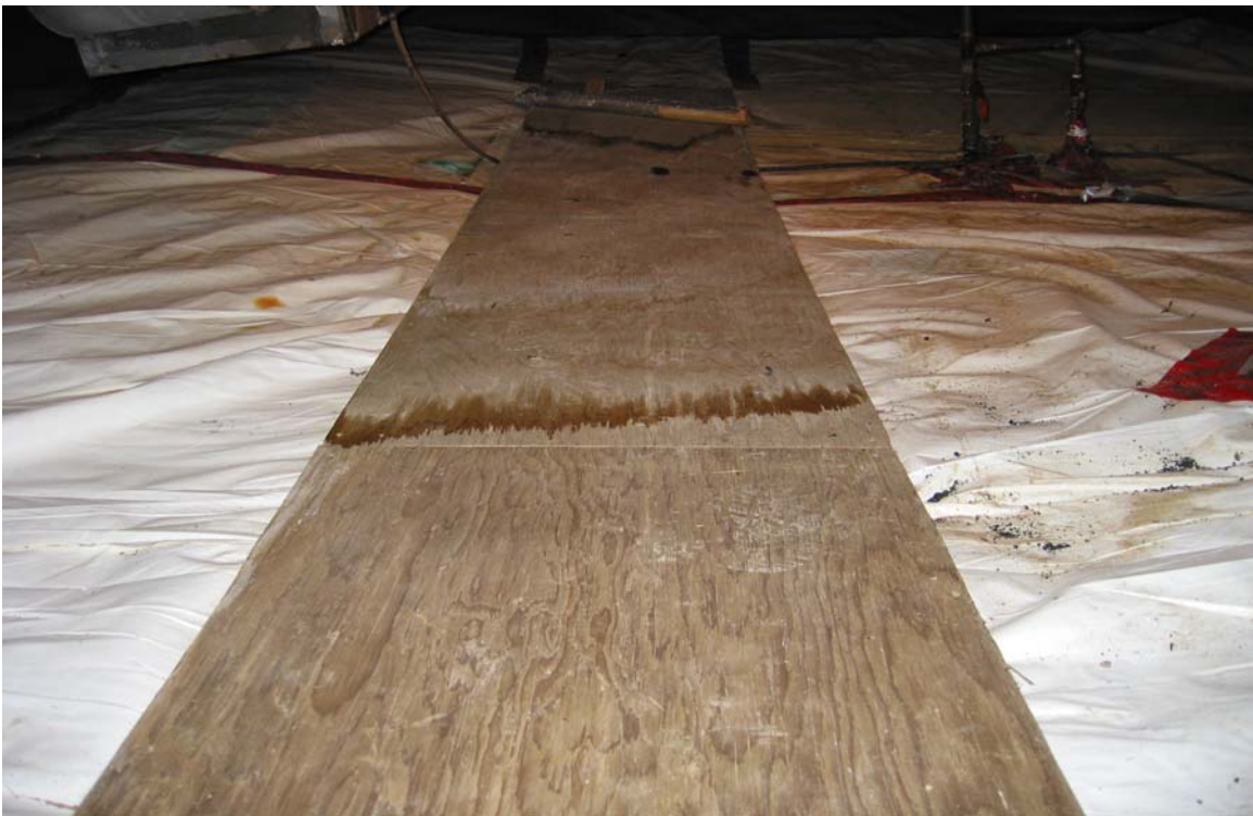
Photo 2: Wood pathways were installed for inspections and maintenance personnel, but are uncomfortable to kneel on and difficult to move for maintenance and cleaning. The floor barrier shows debris and a history of water entry.
