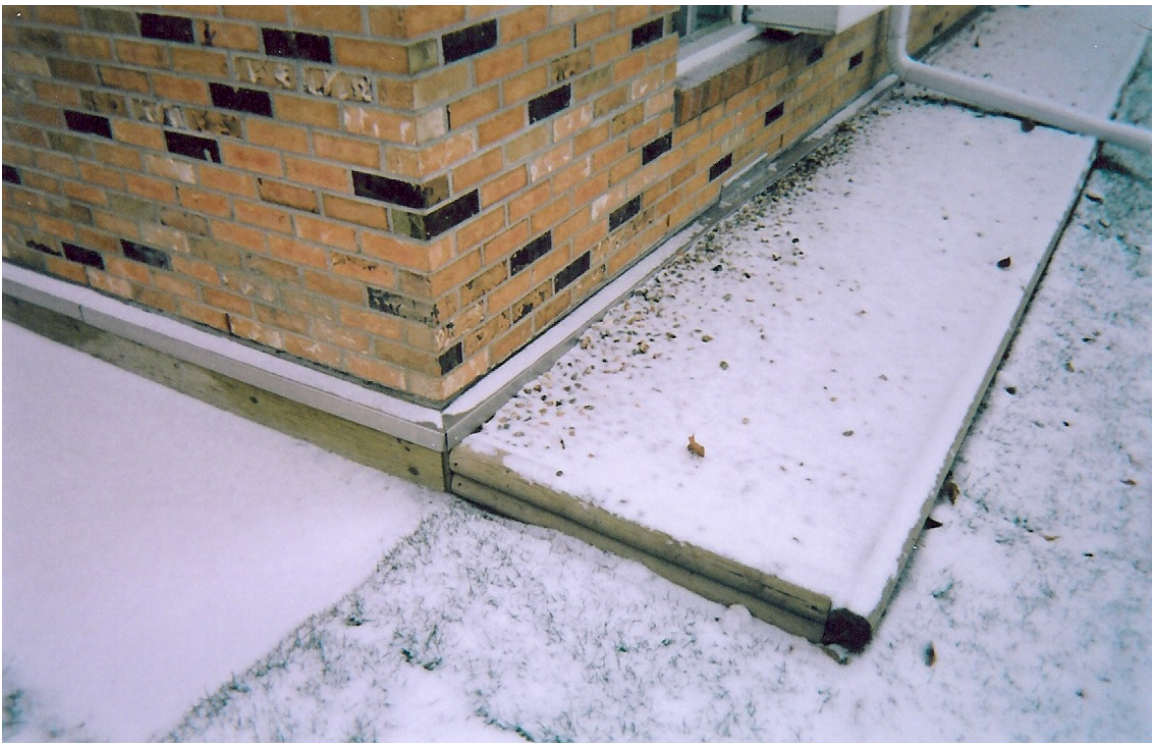
Photo 9: Perimeter of the building has a graded landscape. Exterior walls of the crawl space are insulated from the exterior, covered with pressure treated plywood and capped with metal flashing.
