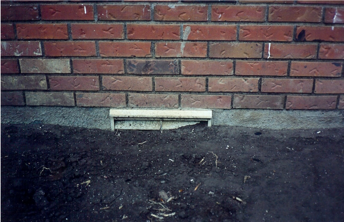
Photo 6: Perimeter of building had poor landscaping. Soil built-up to improve drainage but was above the appropriate level for the building configuration. Ground level vents were open and allowed entry of debris into the crawl space area.
