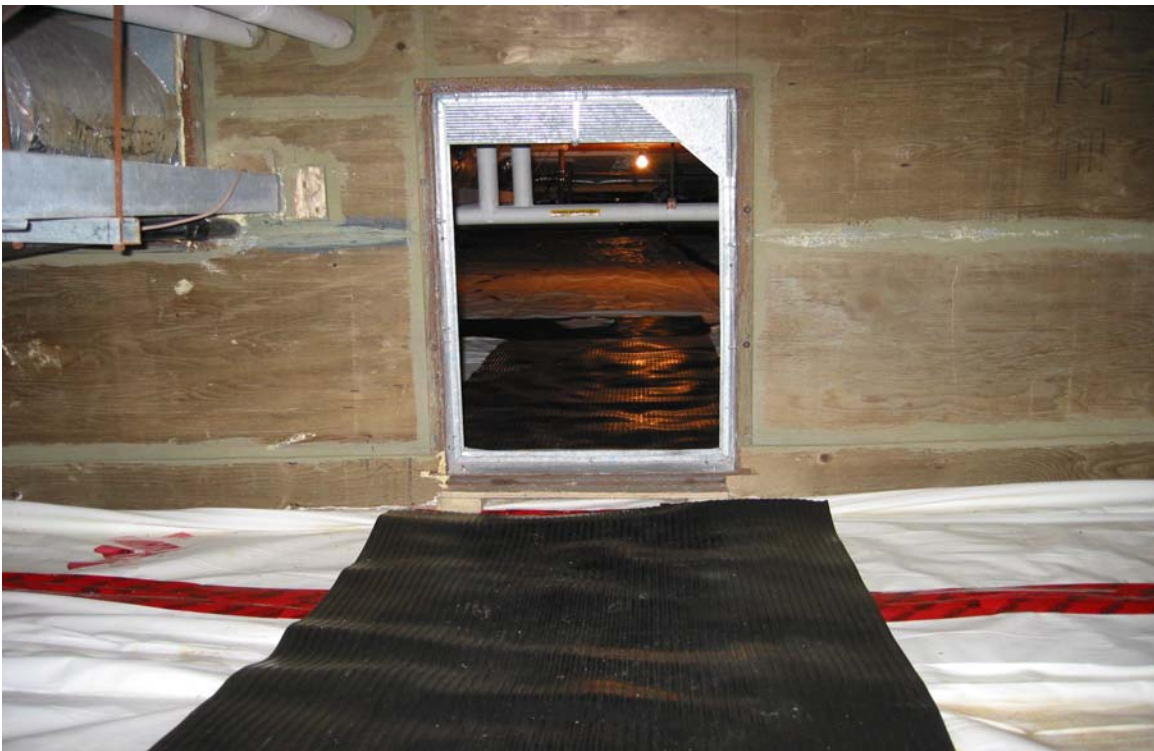
Photo 8: Smoke control walls and fire dampers have been installed to separate various crawl space areas.
