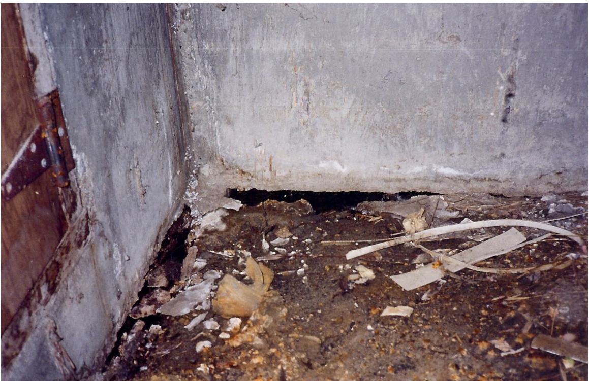
Photo 7: Crawl space floor is sand/gravel. The floor was wet and covered with debris. The “floor barrier”, which consisted of sheets of poly laid around the general floor area, was unsealed and incomplete.
