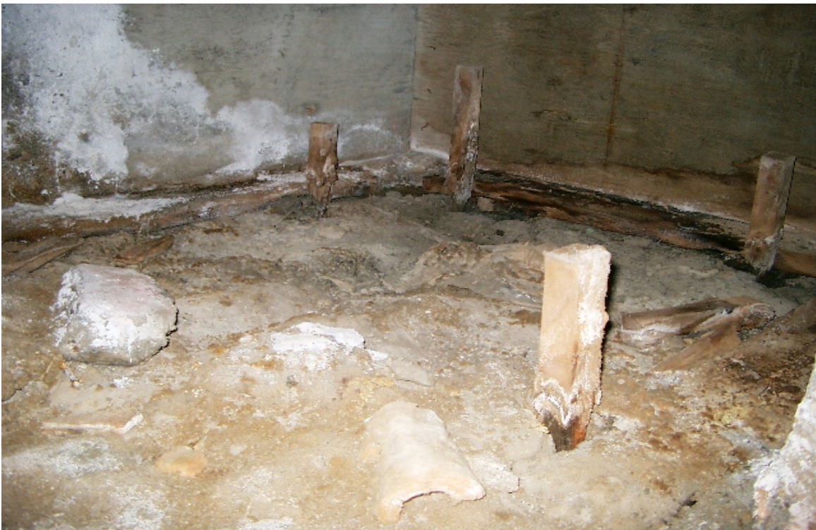
Photo 1: Original crawl space floor showed extensive water damage and deterioration.
