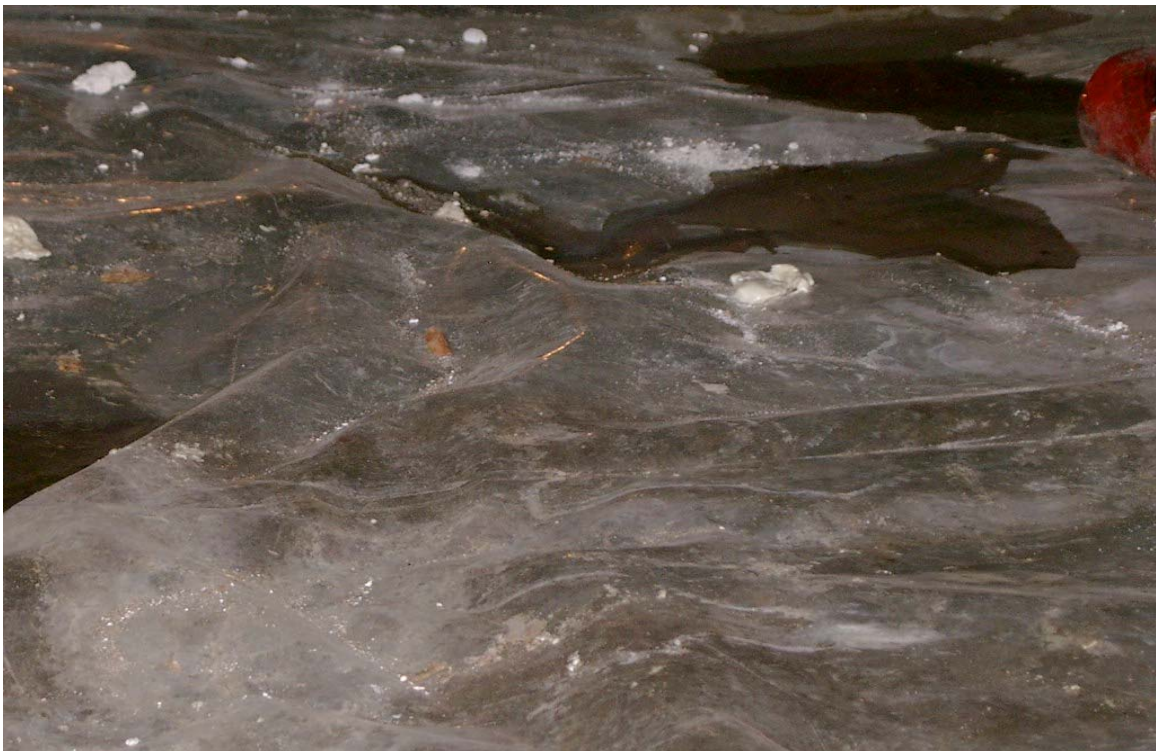
Photo 3: Debris and water were present on the surface of the existing polyethylene floor barrier.
