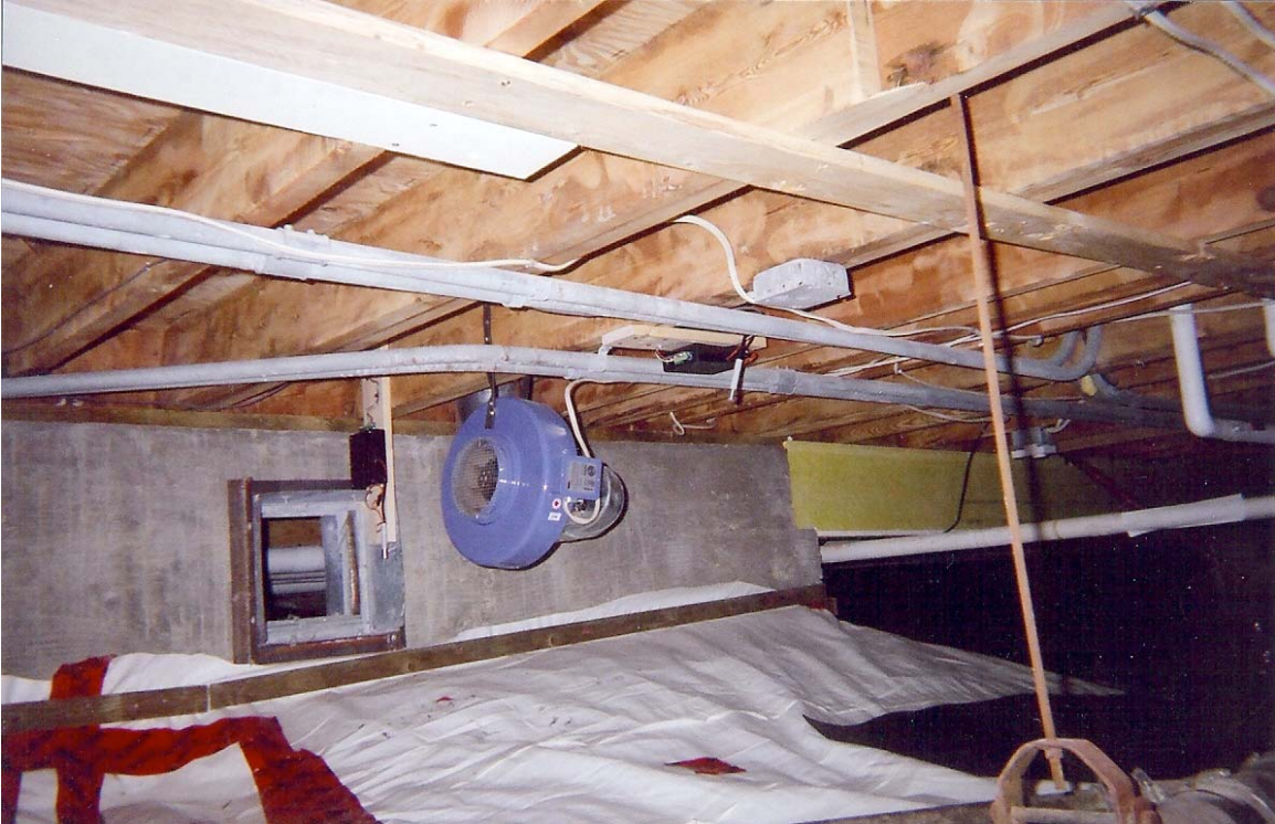
Photo 5: Dedicated crawl space exhaust fan provides a continuous negative pressure relative to the main floor of the facility. Fan discharge is ducted to a roof mounted exhaust hood through well sealed and insulated round metal ducting. Humidiguard™ humidity and temperature reference sensor located downstream of each crawl space zone to assess crawl space environment conditions.
