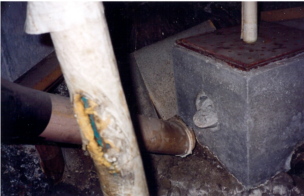
Photo 3: Deteriorated piping. Sump pump piping was disconnected and drained water onto the crawl space floor (note the concrete sump well never had an opening for foundation drainage piping to discharge properly).
