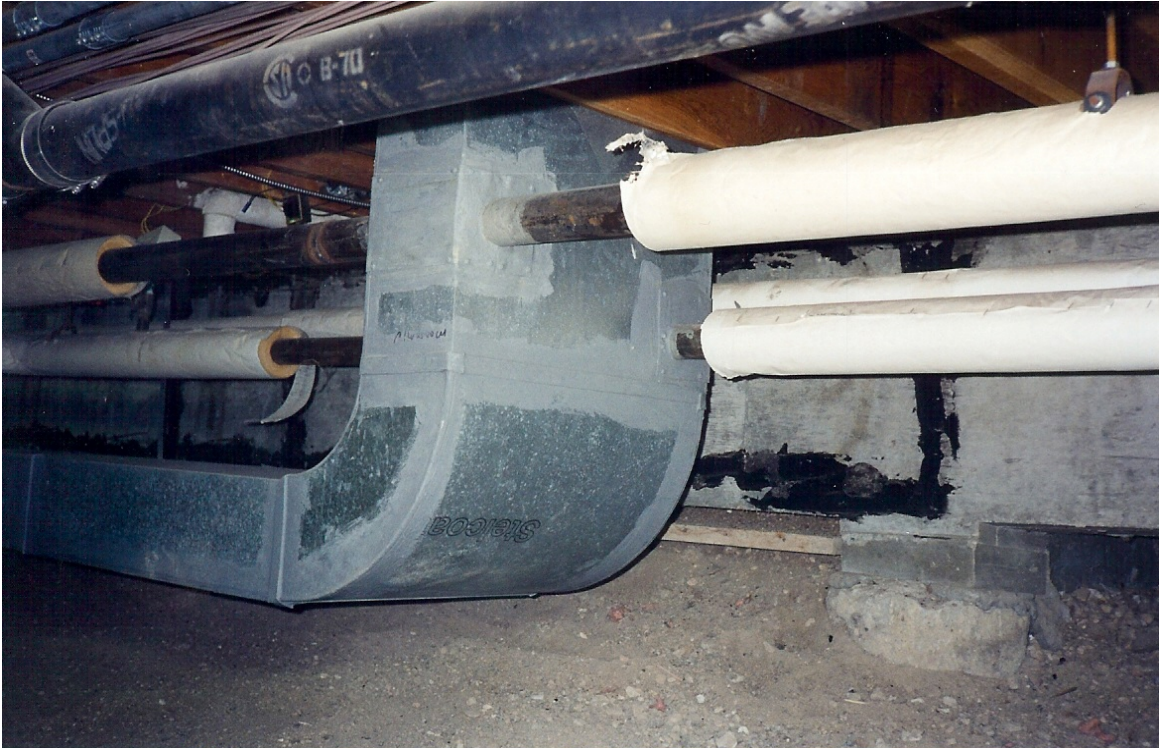
Photo 1: Ventilation ducting in crawl space area. Non-insulated sections of piping. Duct sealing was conducted as a final step in sealing and isolating the crawl space before other remediation was initiated.
