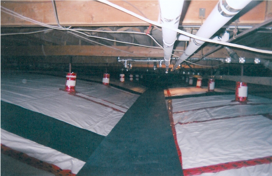
Photo 8: Clean, durable crawl space floor. Floor barrier is sealed at all connections and extends up the concrete piles. Black rubber floor mats provide floor barrier protection and are easily moved/removed for cleaning.
