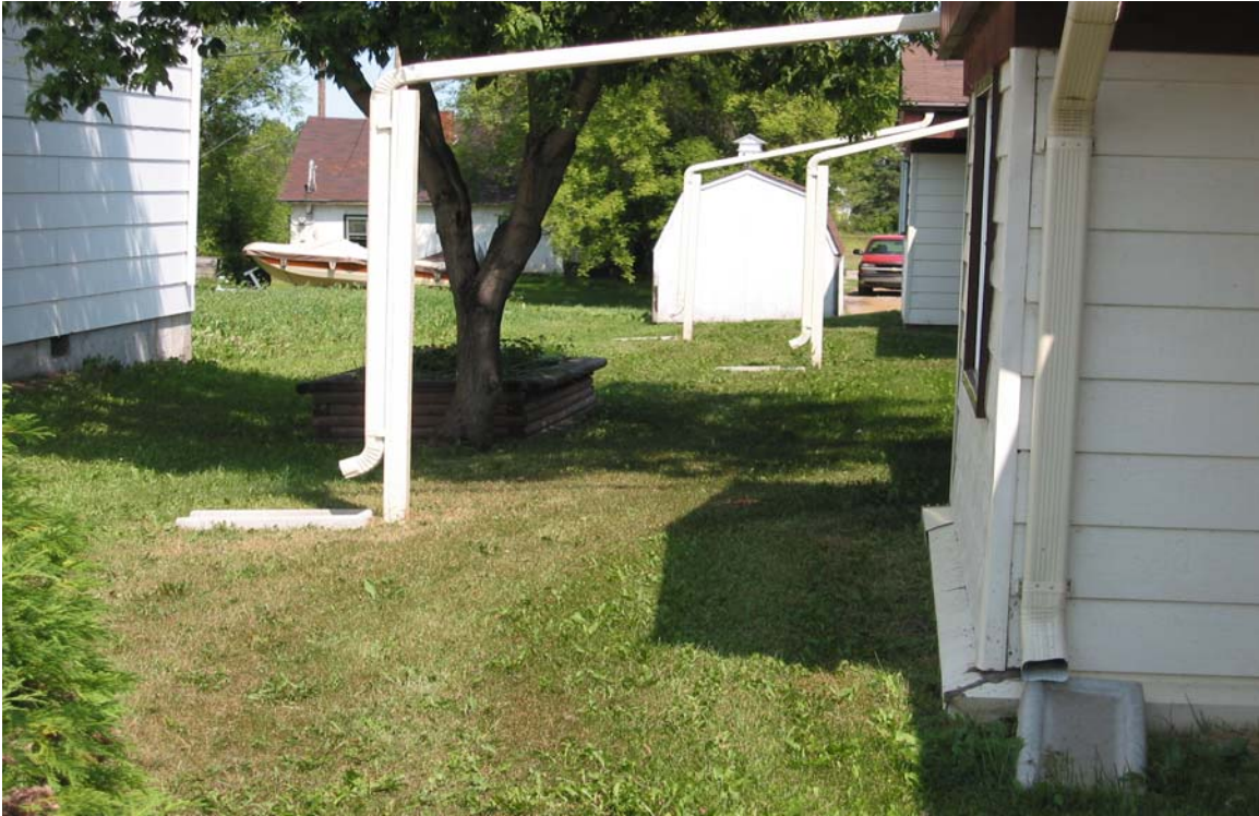
Photo 9: Landscaping and proper downspout attachments have prevented external water entry into the crawl space.
