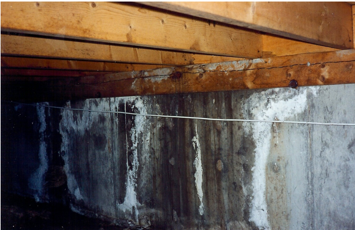
Photo 5: Exterior concrete wall of the crawl space was dirty and stained. Extensive mineral deposits indicated chronic water entry. The wood joists were moldy and deteriorated.
