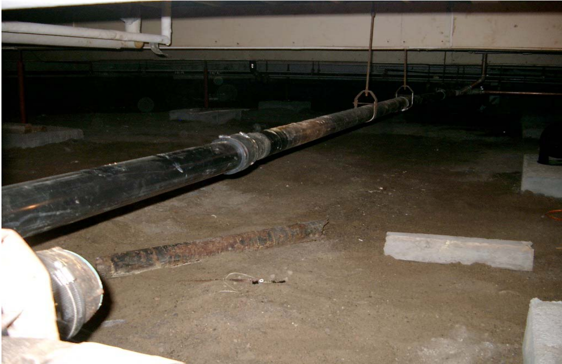
Photo 2: Debris (including garbage and deteriorated piping) was on the crawl space floor. In many areas, no floor barrier was present and the exposed sand/soil floor was damp.
