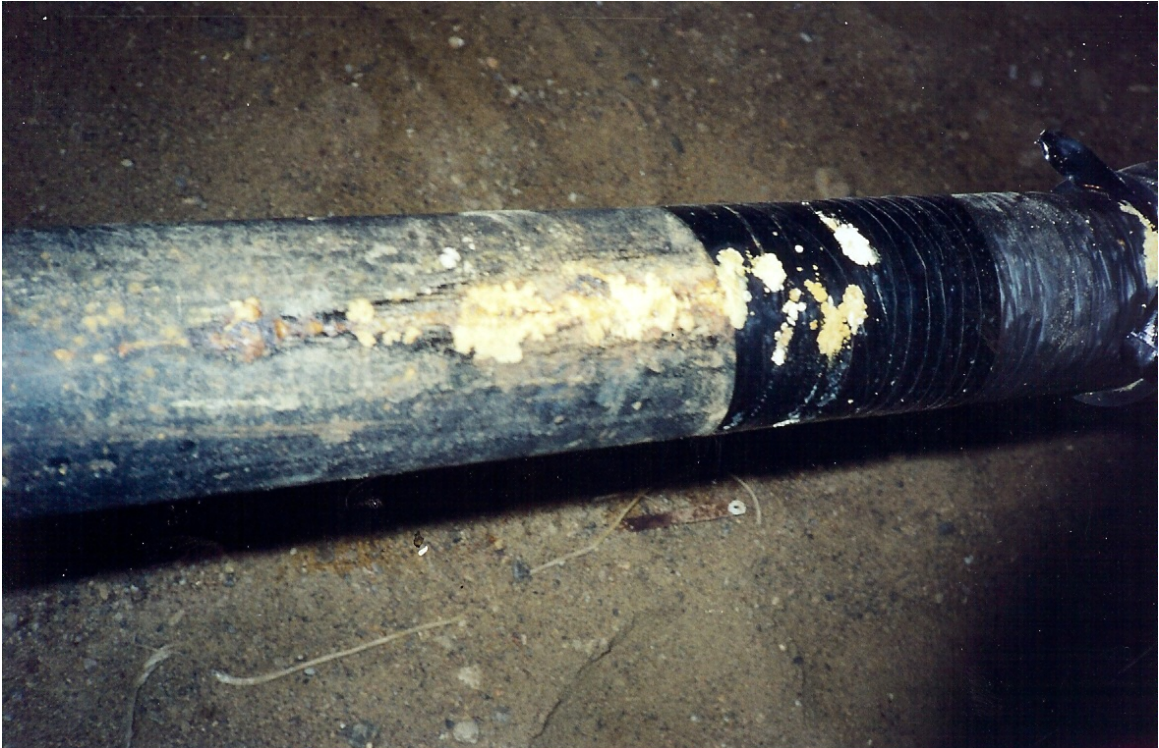
Photo 2: Longitudinal crack in the sewer piping in the crawl space area (repaired by wrapping with electrical tape).
