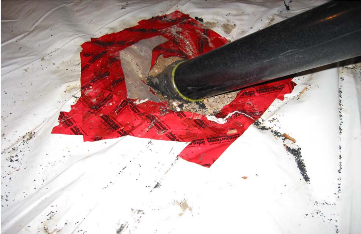
Photo 1: Floor barrier surrounding a new piping installation has not been sealed. Debris from the installation has not been removed and is scattered on the floor barrier.
