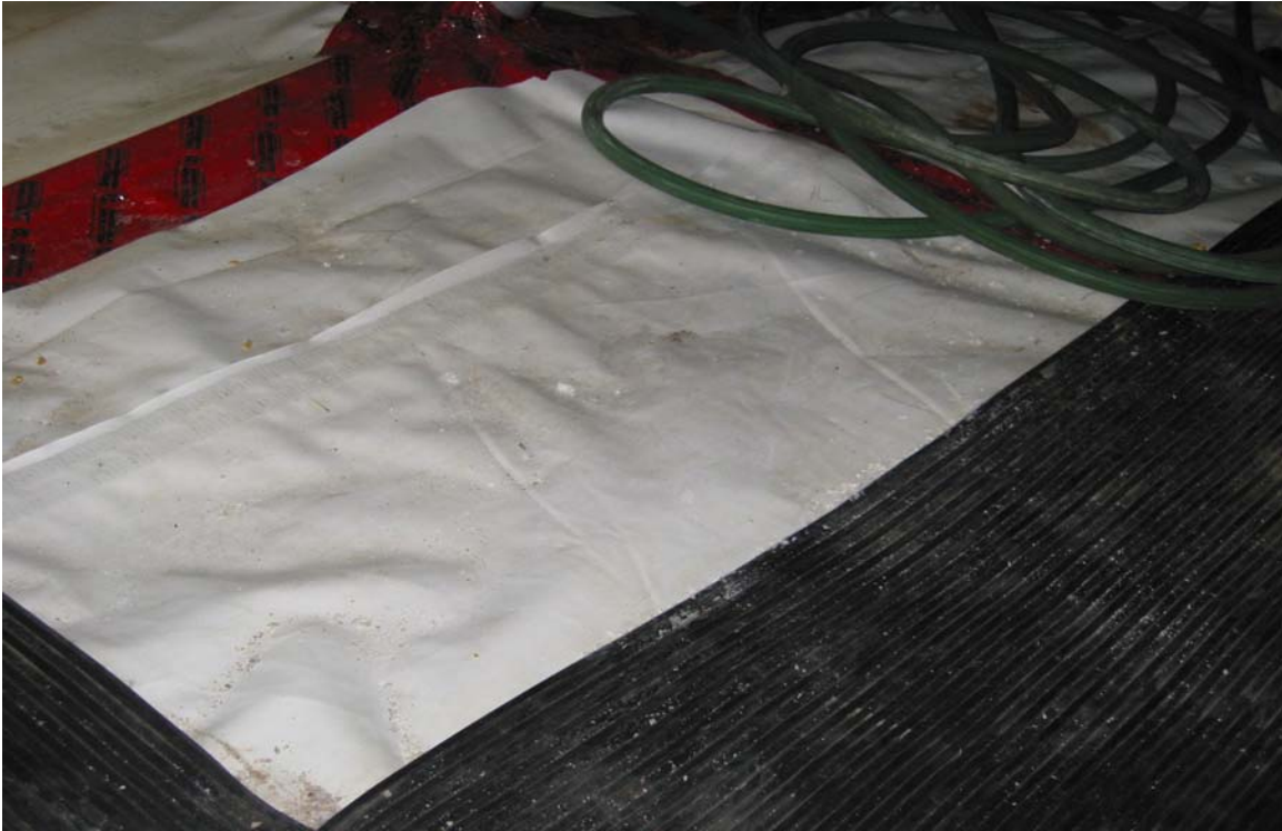
Photo 3: Crystallized bleach remains on the crawl space floor barrier from the bleaching method used for mold removal.
