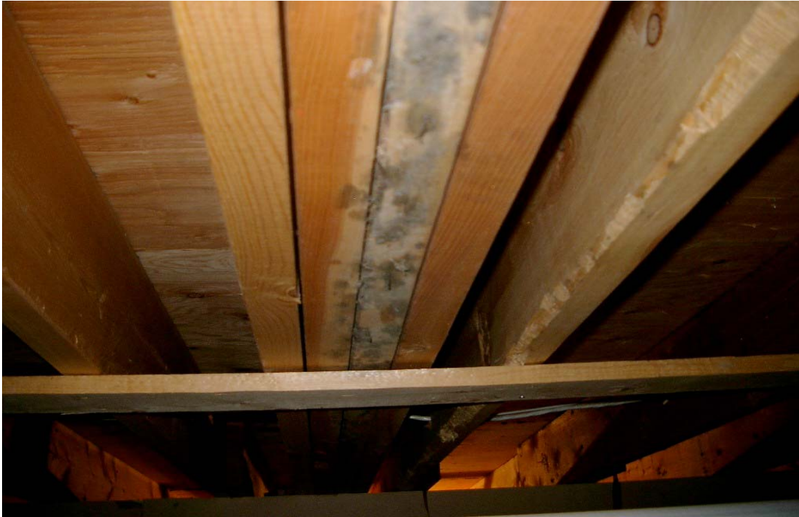
Photo 4: Mold was visible on some of the wooden components within the crawl space area.
