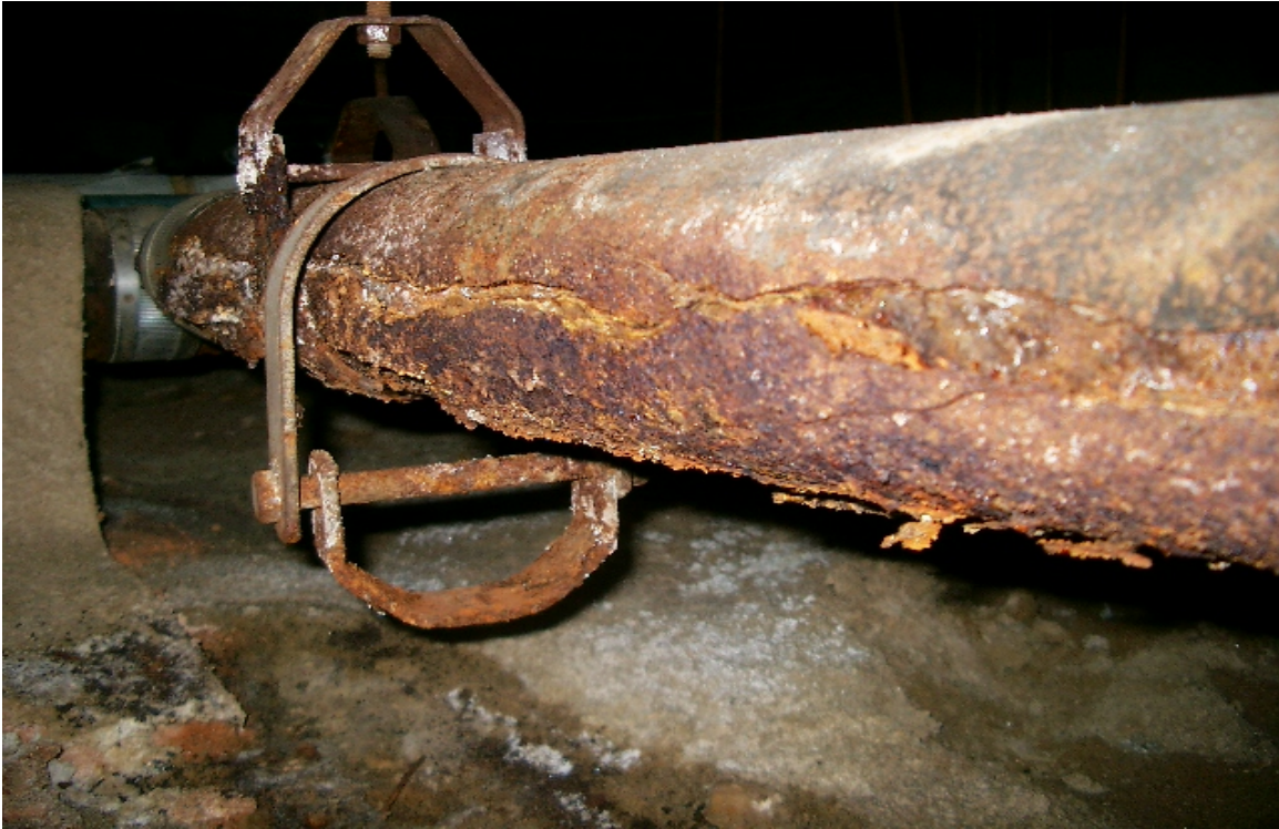
Photo 8: Old, corroded piping was the source of some water entry into the crawl space.
