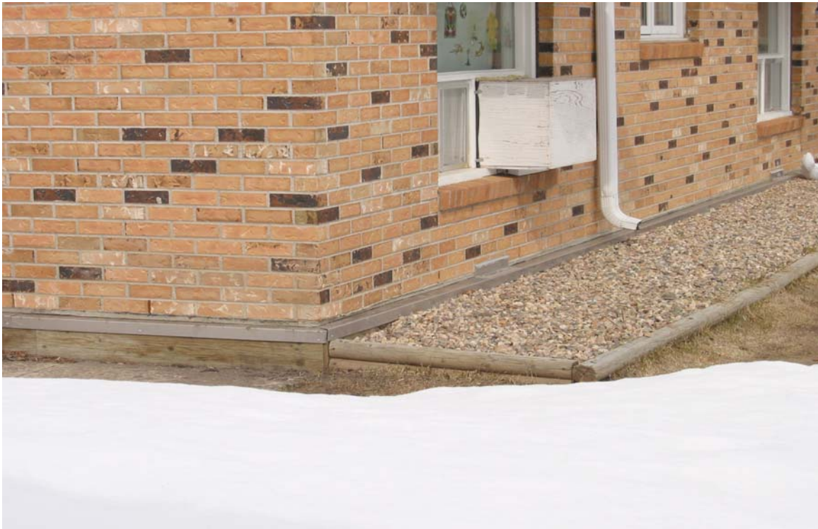
Photo 8: Exterior insulation and metal flashing are in good condition. The exterior landscaping and downspouts have been helpful in keeping water away from the crawl space exterior.
