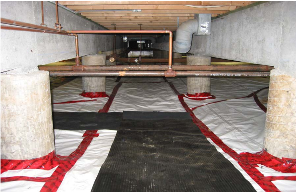
Photo 4: Crawl space floor barrier and tape is in good condition. The installed rubber floor mats, which can be moved for cleaning and maintenance, are useful in enhancing the durability of the floor barrier.
