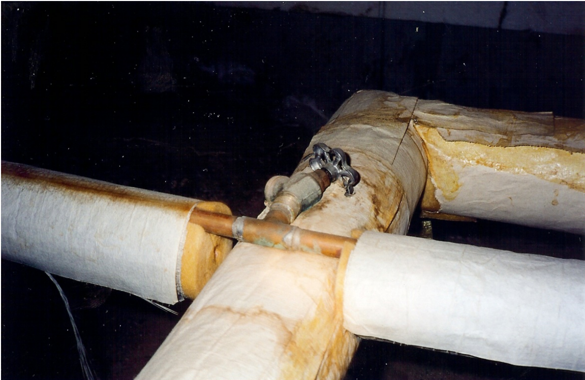
Photo 1: Deteriorated, leaking plumbing and piping in the crawl space.
