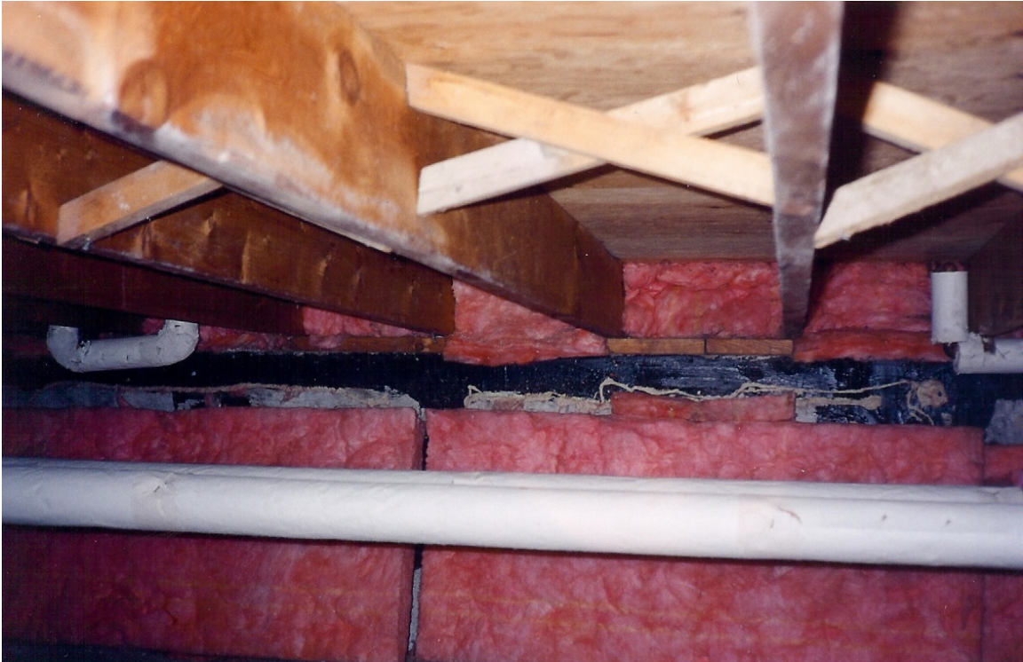
Photo 3: Interior batt insulation on the exterior walls of the crawl space was not sealed or covered. Floor joists are visibly moldy.
