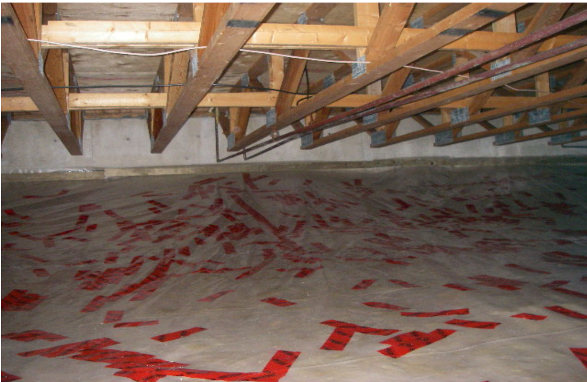
Photo 6: Sections of the poly floor barrier have required extensive patching to repair punctures and tears.
