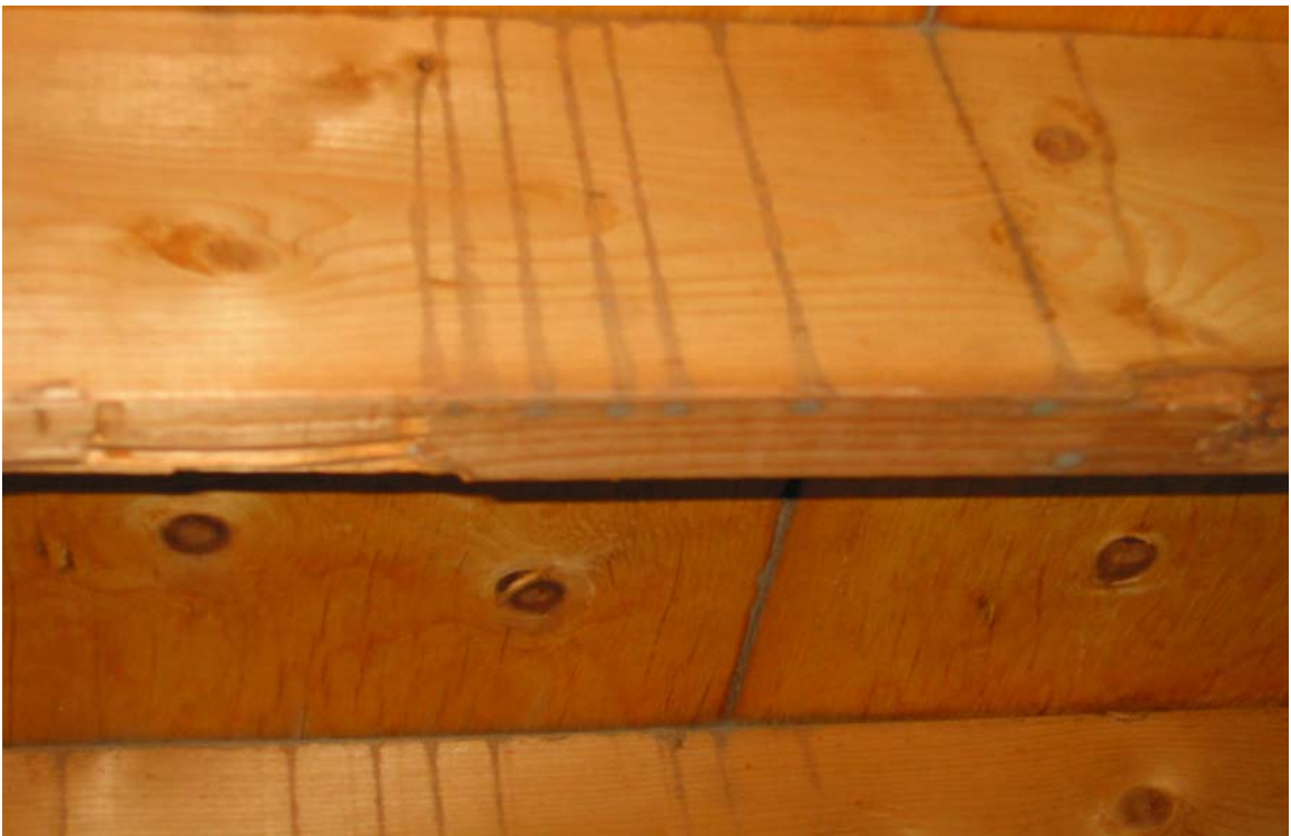
Photo 11: Some floor joists show signs of staining, which is most likely residual bleach.
