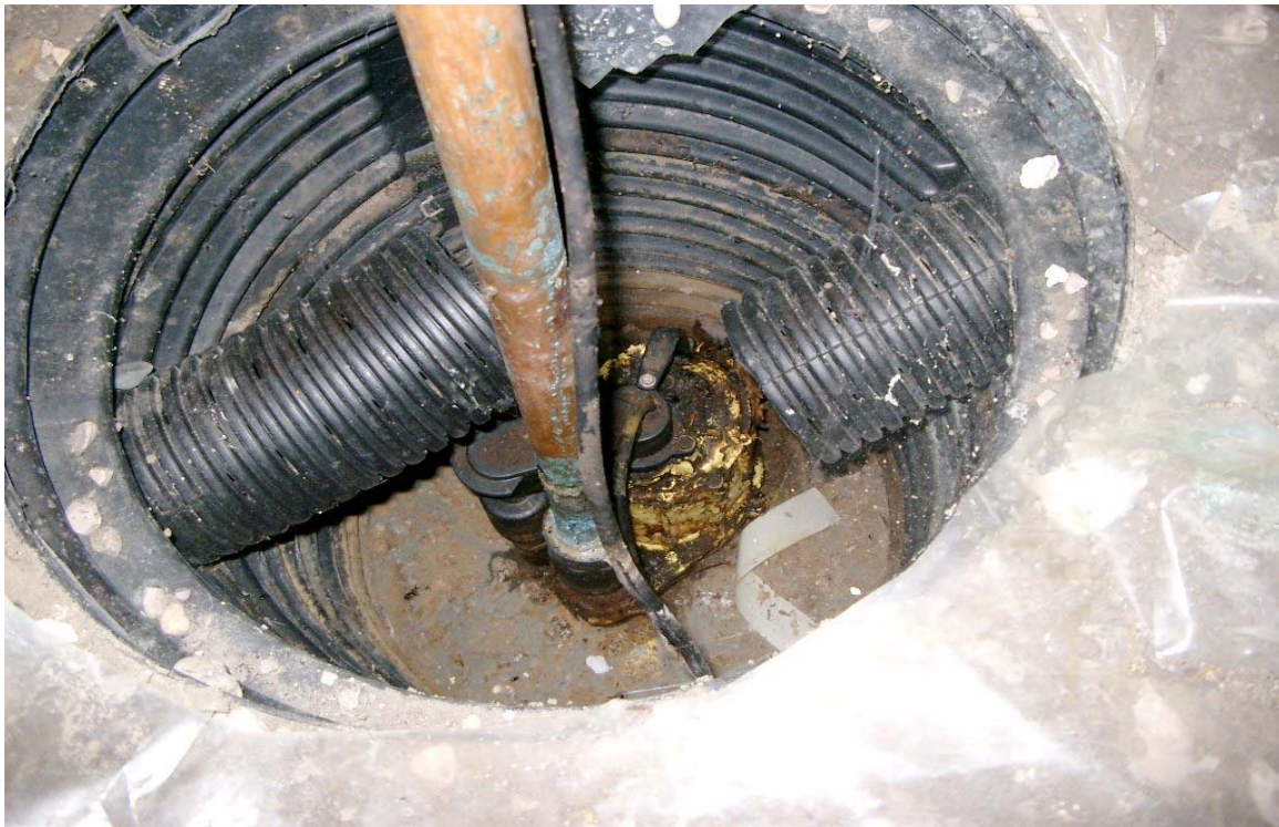
Photo 1: Existing sump pump was dirty and rusted and was not covered or sealed.
