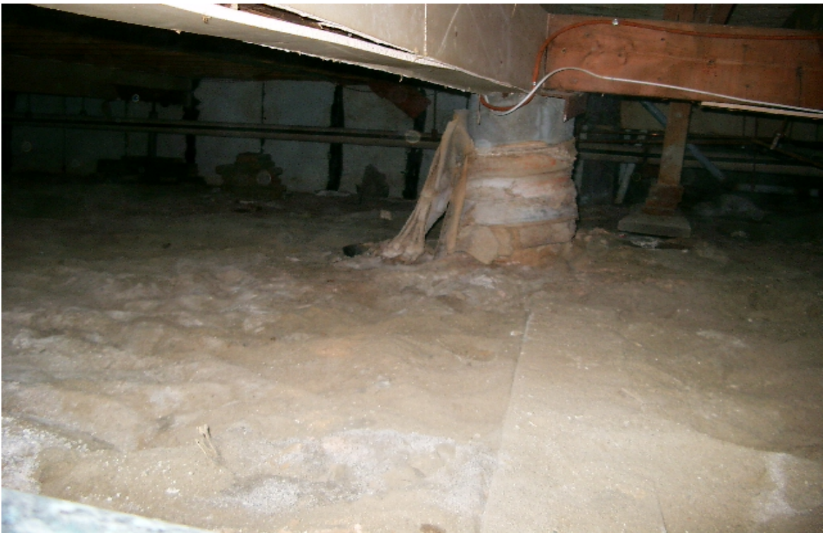
Photo 5: Crawl space floor is sand/gravel. Concrete piles were wrapped in deteriorated paper.
