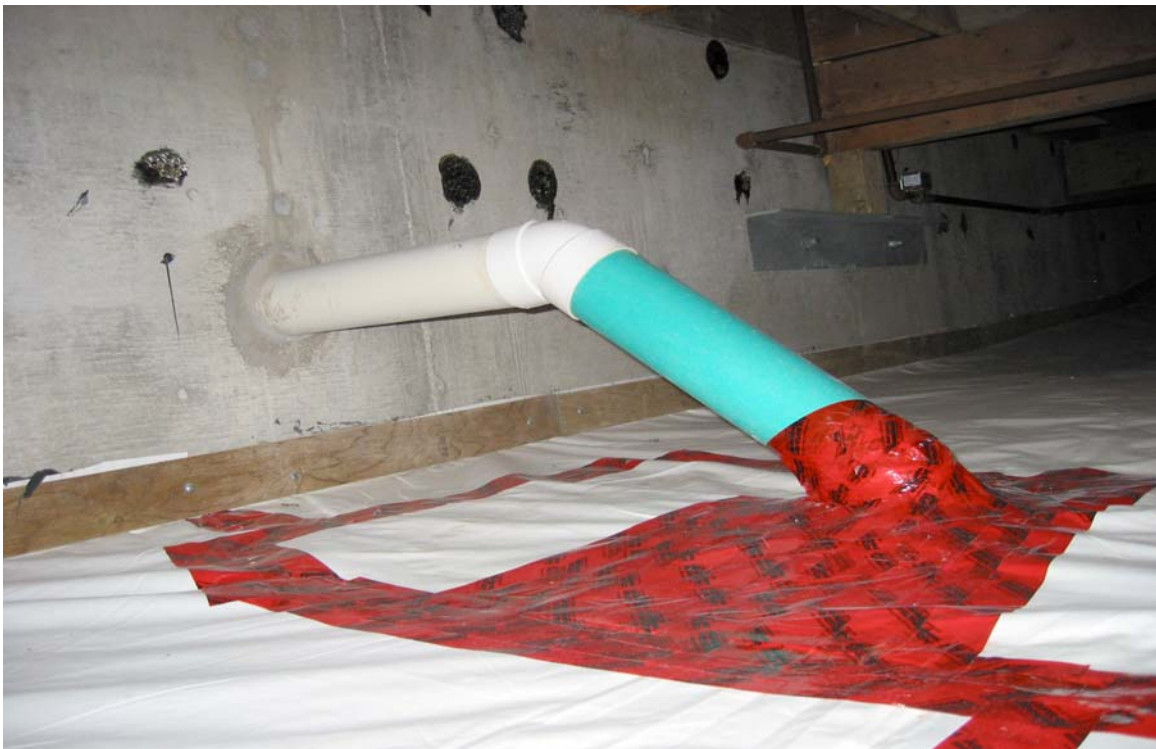
Photo 9: Floor barrier is well attached to the exterior walls and is sealed around all columns, piping and other floor barrier penetrations.
