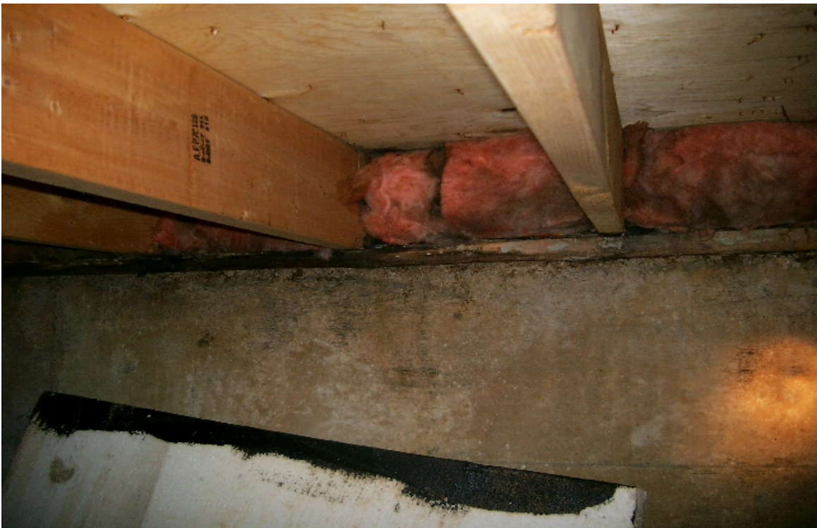
Photo 3: Exterior walls were insulated from the interior side of the crawl space. Joist ends were moldy and deteriorated.
