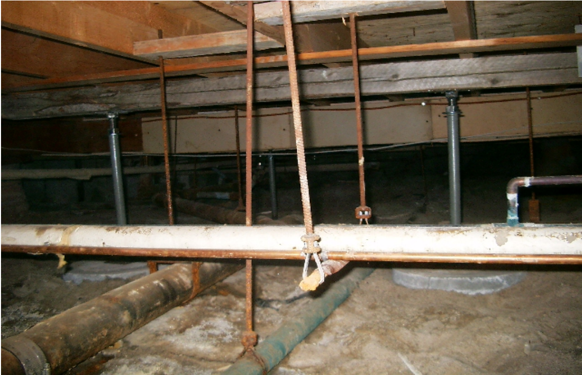
Photo 6: Old, corroded piping within the crawl space area.
