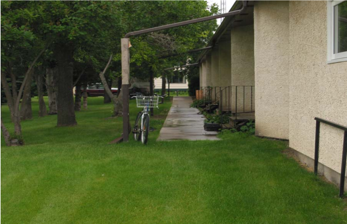
Photo 5: Landscaping around the building has been modified to move water away from the building perimeter.
