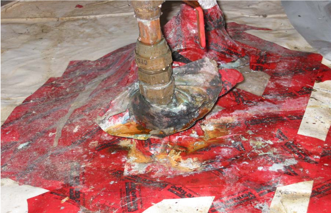
Photo 3: Extensive sweating on cold water pipes has caused stains on the floor barrier and has affected attachment of the tape.
