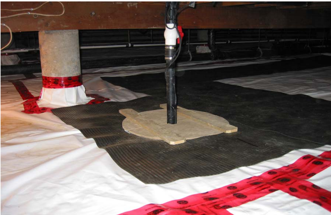
Photo 13: New sump pump installed at a low point in the crawl space.
