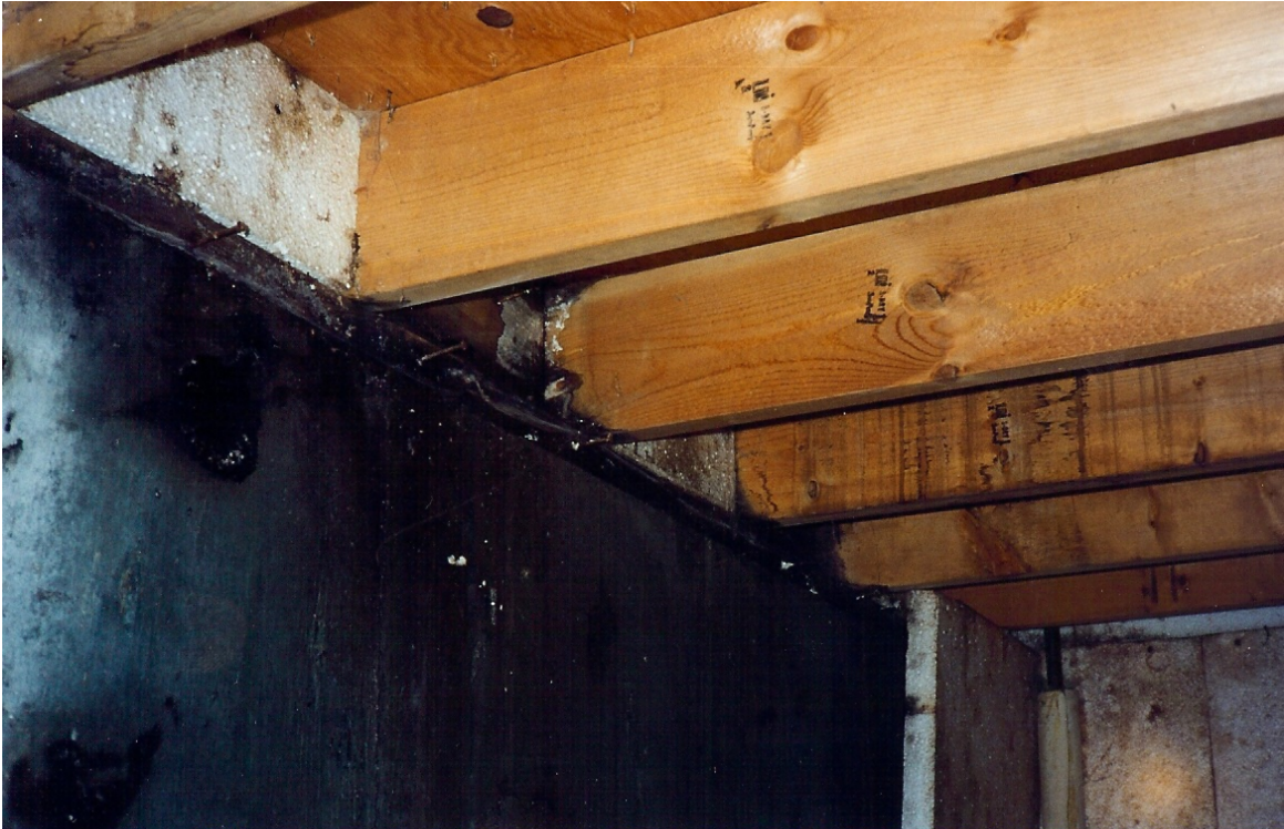
Photo 4: Ends of the rim joists were rotten, moldy and deteriorated. Bead board insulation was present on the interior side of the exterior walls in the crawl space. The insulation was poorly installed, the edges were not sealed and many sections were missing.
