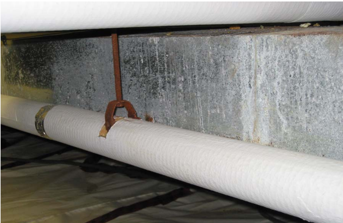
Photo 2: Bleaching of the wood joists has caused damage to the galvanized metal ducting within the crawl space area.
