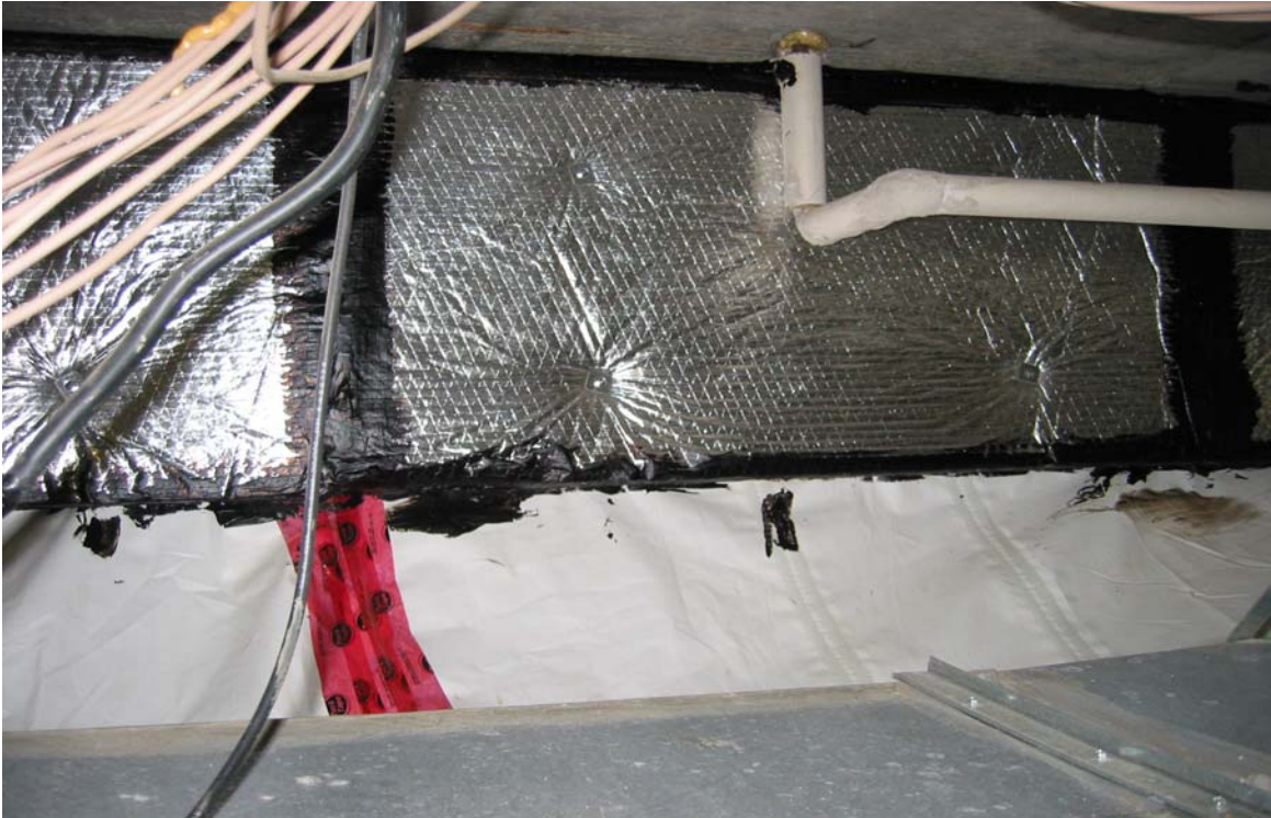
Photo 7: Exterior foil faced wall insulation is in good condition.
