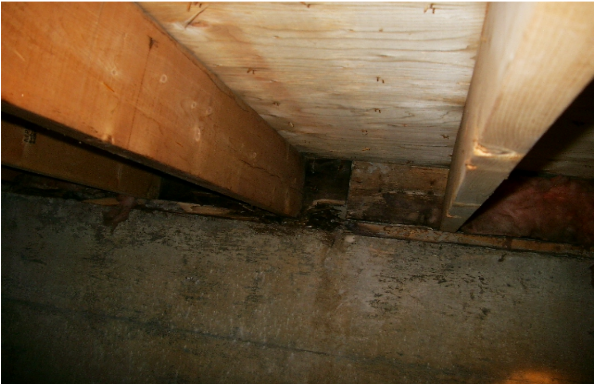
Photo 7: Visible mold and deterioration on the rim joists and ends of the floor joists.
