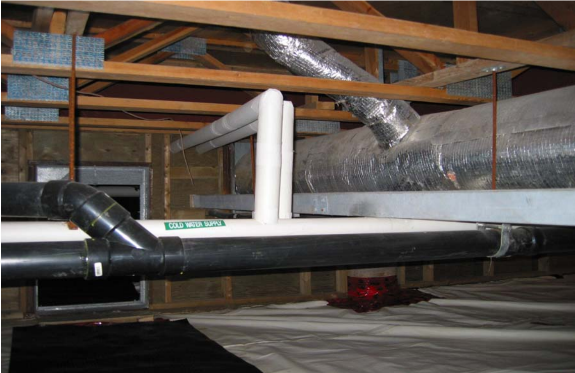
Photo 7: New plumbing, piping and ventilation equipment has been suspended above the floor barrier. The insulation around piping and ducting is well sealed and in good condition.
