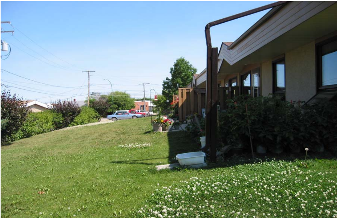
Photo 6: Exterior landscaping and downspouts have been effective in moving water away from the exterior of the building.
