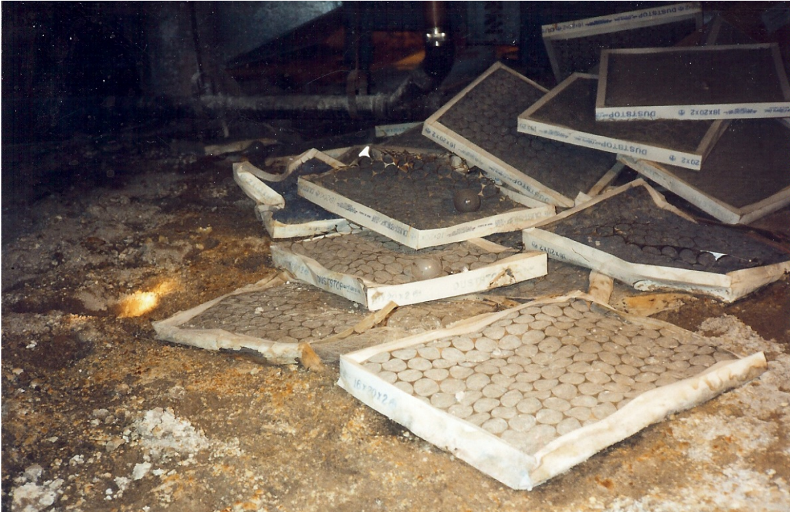
Photo 3: Dirty, moldy furnace filters, along with light bulbs and pieces of insulation, were on the dirt/sand crawl space floor.
