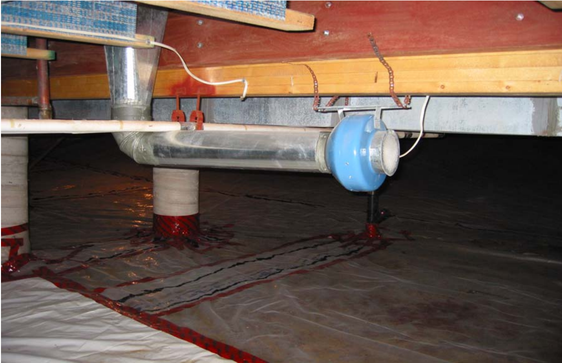
Photo 7: The crawl space has a dedicated exhaust fan installed to provide a continuous negative pressure in the area relative to the main floor. The fan discharge is ducted to a roof mounted exhaust hood through well sealed and insulated round/rectangular metal ducting.
