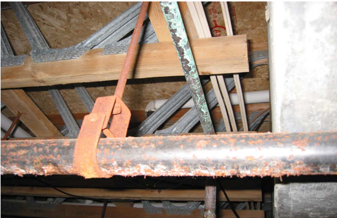
Photo 6: Rust is present on many of the crawl space piping components as a result of the use of bleach for mold removal.
