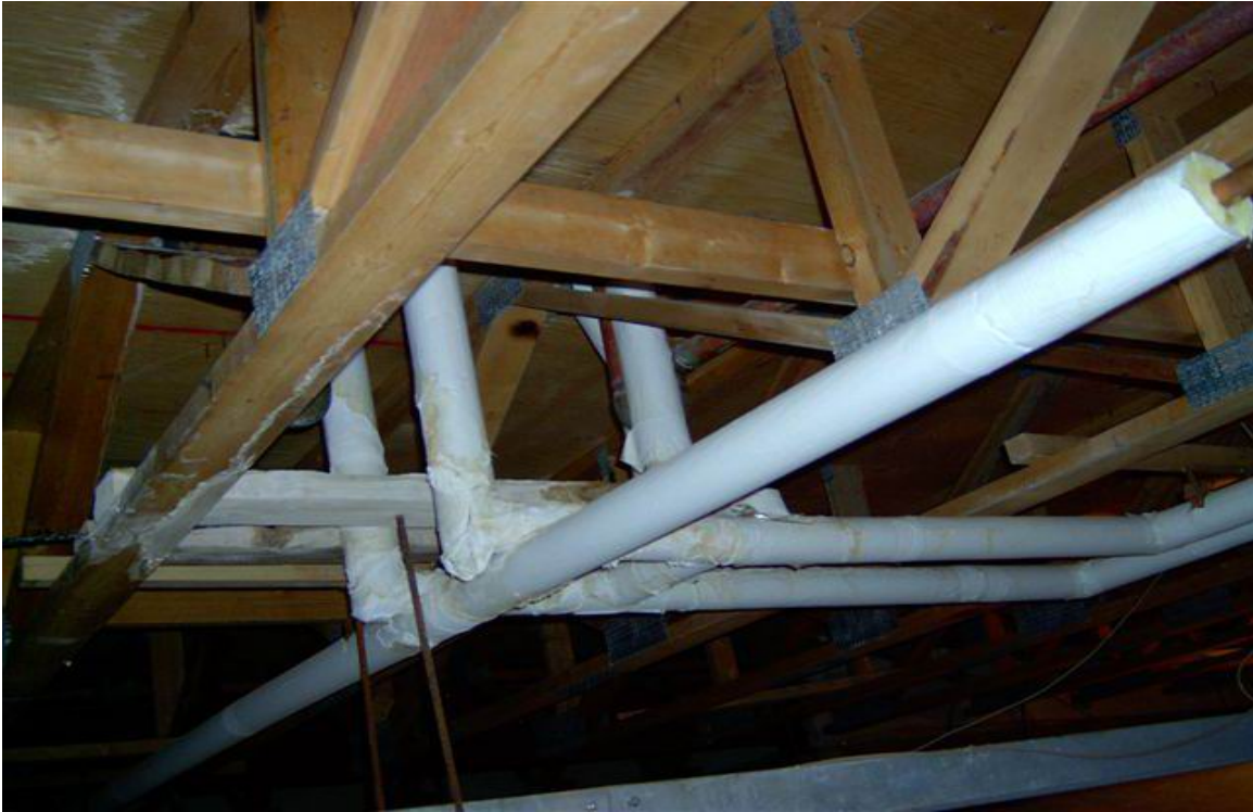
Photo 1: Water markings and staining are visible on the wooden components in the crawl space area. The pipe insulation also shows evidence of water damage.
