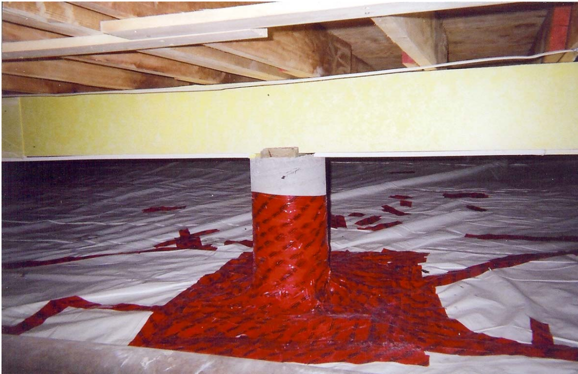
Photo 6: Floor barrier is in good condition and tape is well attached. Concrete piles are wrapped to provide a continuous barrier between the crawl space area and the soil. Densglass Gold™ gypsum fireguard installed on main built up beams.
