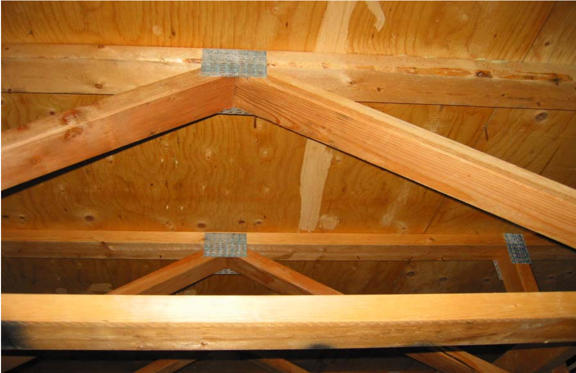
Photo 5: Trusses are in excellent condition with no signs of mold re-growth.
