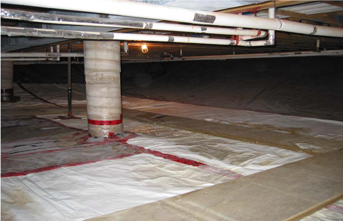
Photo 5: The floor barrier, with the exception of the stains and specifically damaged areas, is in good physical condition. The floor barrier is a mixture of Permalon™ and polyethylene.
