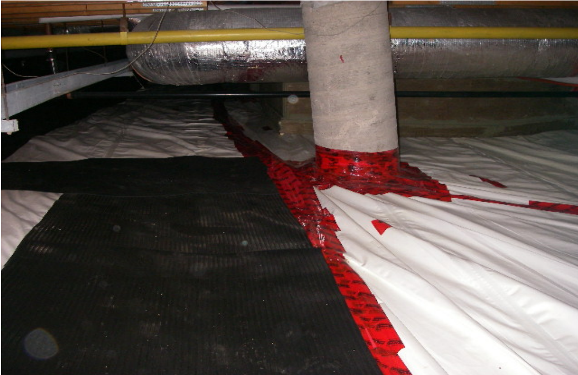
Photo 4: The Permalon™ floor barrier and tape are in good condition and have not required significant repairs (see photo 6). The floor barrier extends up concrete piles and is sealed around each column.
