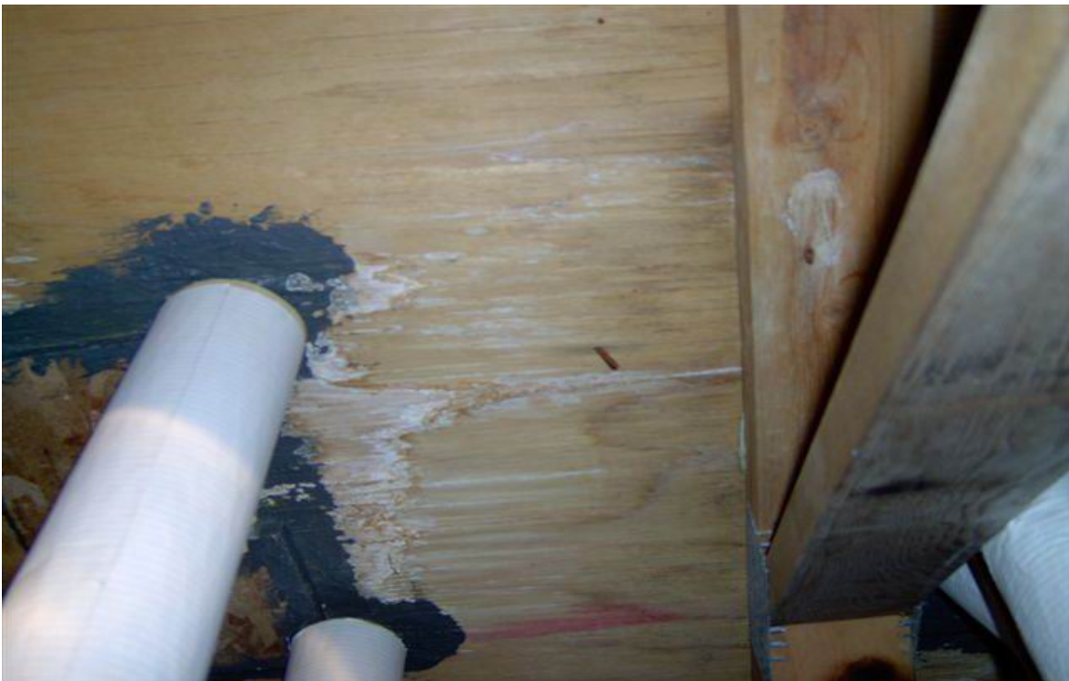
Photo 2: Water markings are visible on the subfloor and trusses.
