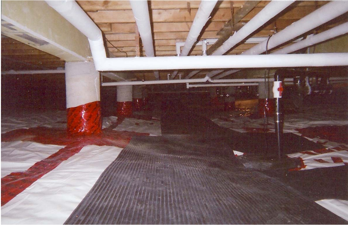
Photo 8: Rubber mats provide a pathway for maintenance personnel. Sump pumps are covered and sealed and are functioning properly. Piping is suspended off the floor and the pipe insulation is in good condition.
