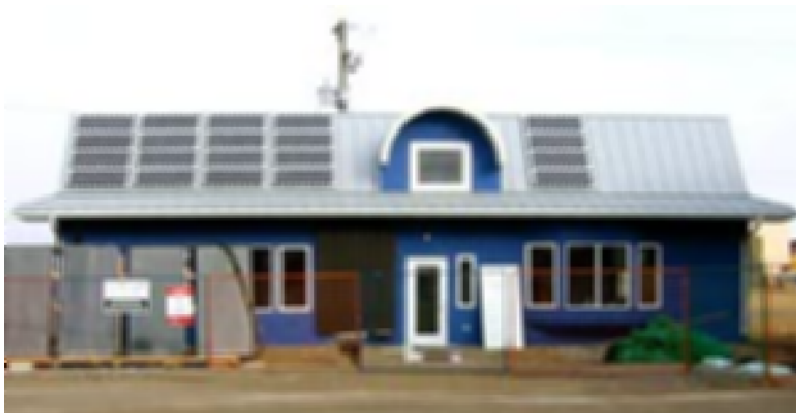
Airdrie Recycling Centre, 2kW rooftop PV installation. Airdrie, AB (photo source: ASH Consulting)
