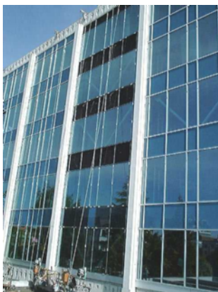
BC Ministry of Health, Pandora Wing of the Blanchard Building BIPV Curtain Wall Installation, Victoria BC (photo: Gordon Howell)
