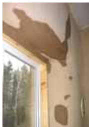
Wet walls from roof leaks (215)
