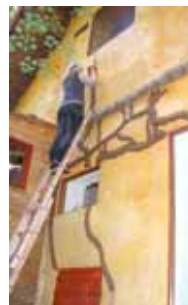
Cracks in earth plaster caulked with cob.
