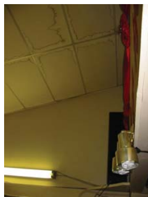
Water Damaged Ceiling
