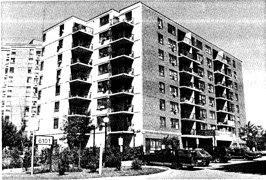
Figure 21: View from the street
