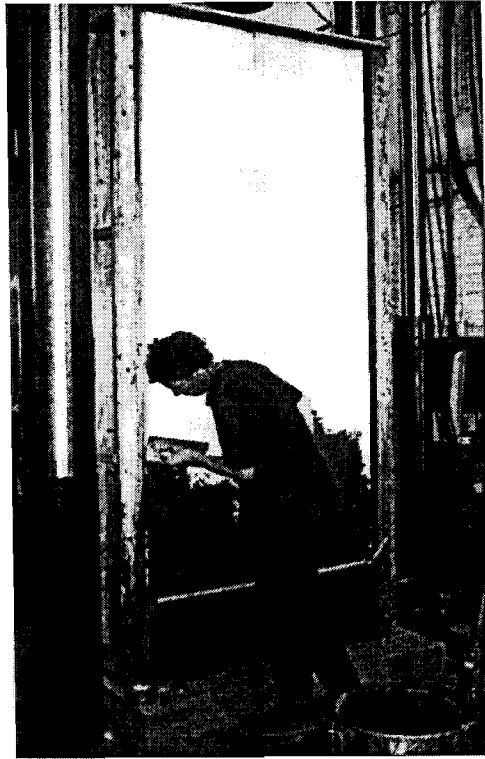
Photo 15: Application of first coat of cement on EPS core
