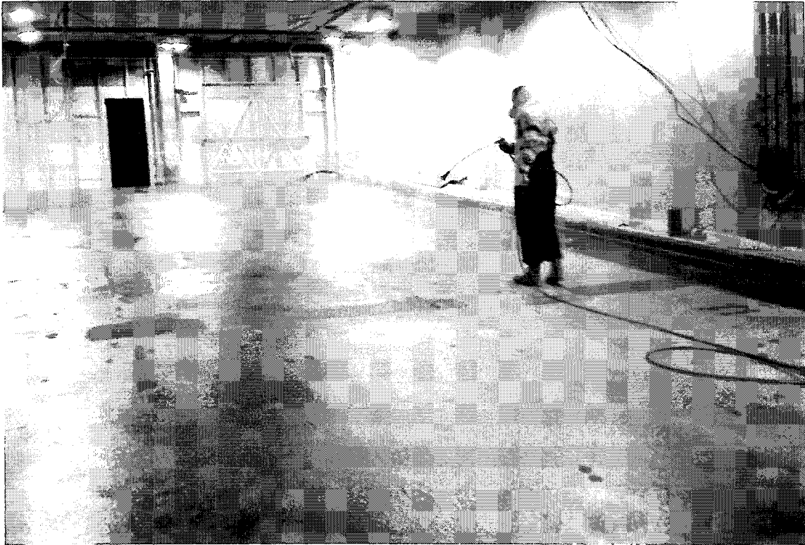
Photograph 5. Application of primer by spray at Ottawa City Hall.
