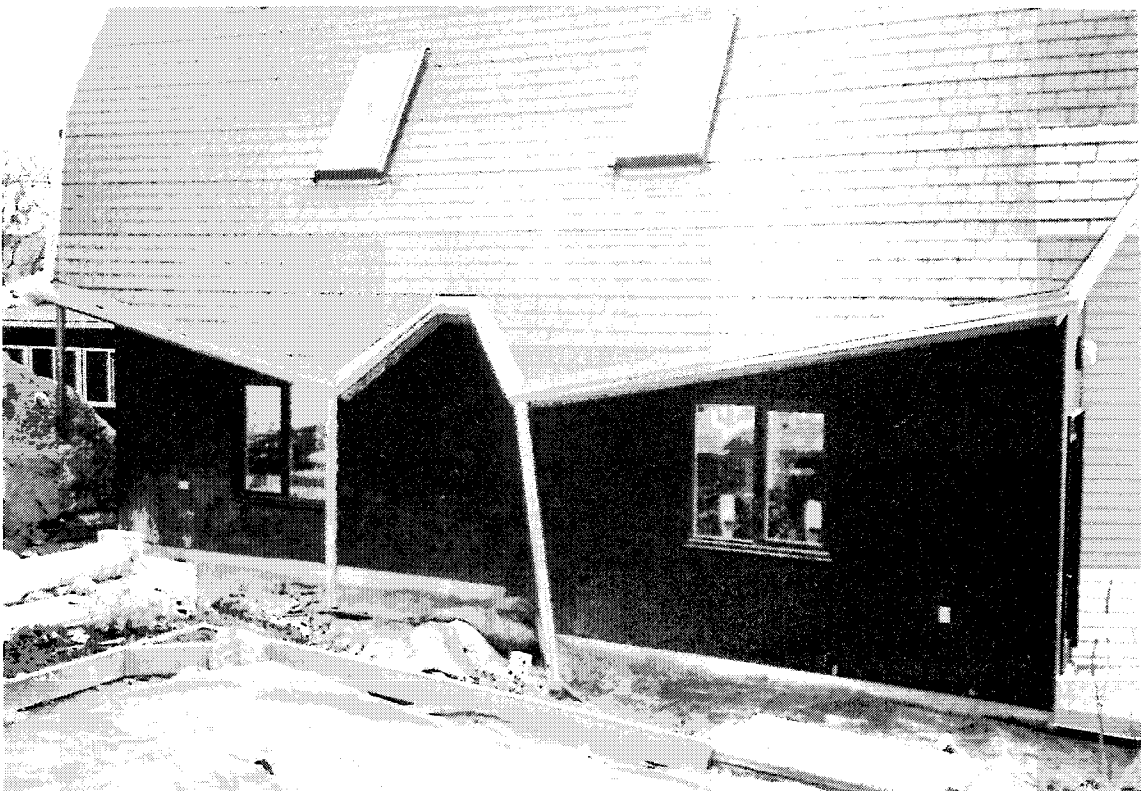
1-2 REAR SLOPING RAIN COLLECTION ROOF
