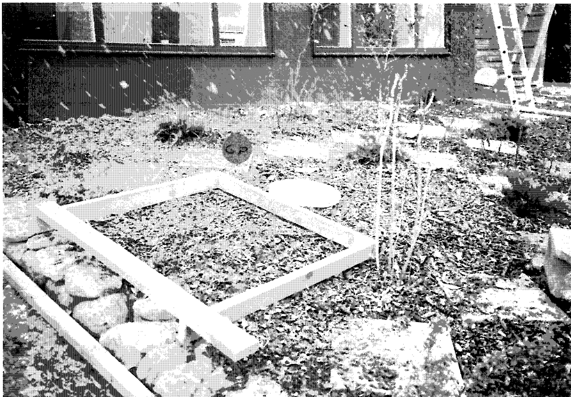
PHOTO 1-24 BURIED WASTEWATER GRAVEL PACK (UNDER THE PATIO STONES NEAREST THE FRONT WALL)
