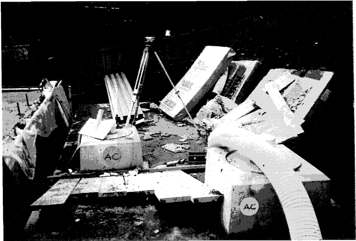
PHOTO 1-5 CISTERN ACCESS CHAMBERS
