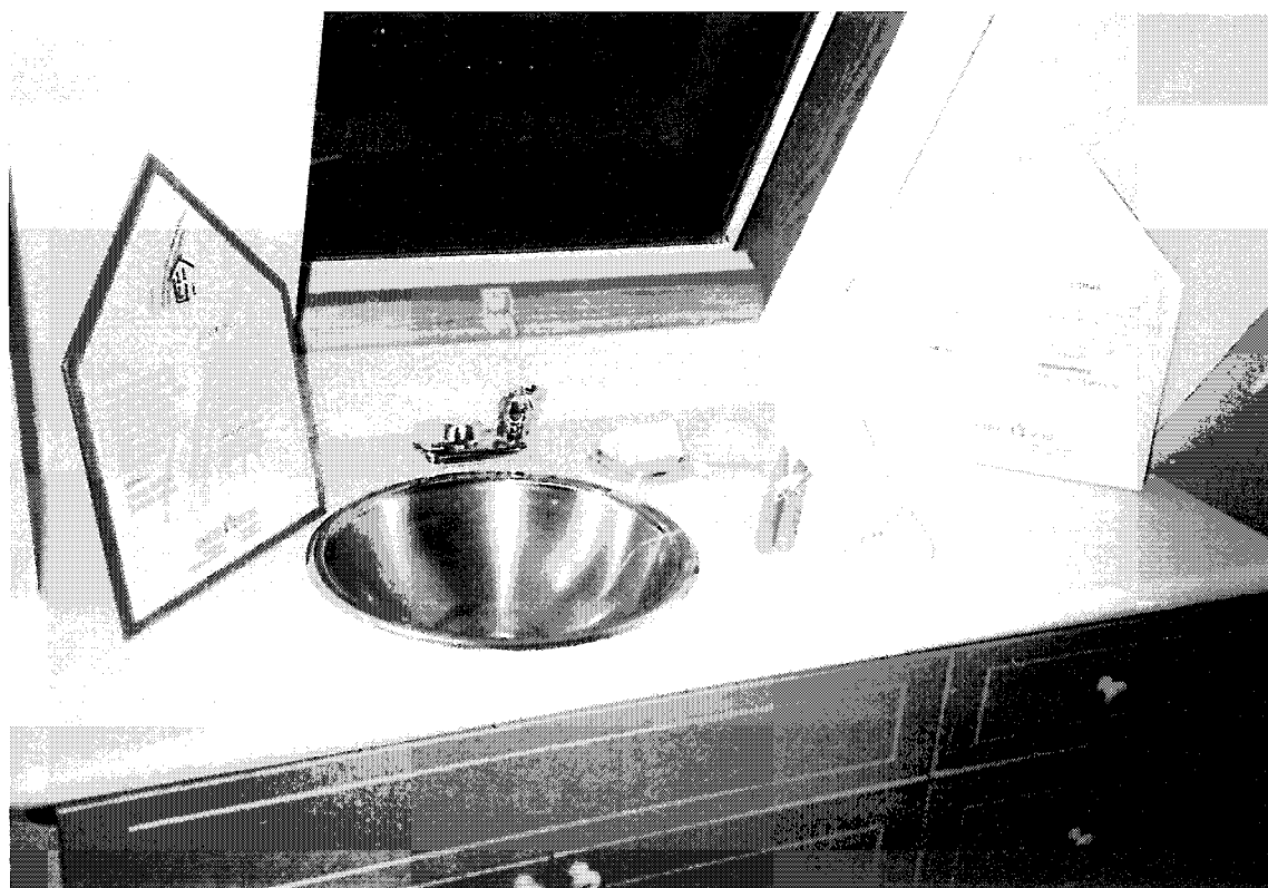
PHOTO 3-2 WATER CONSERVATION FIXTURES
