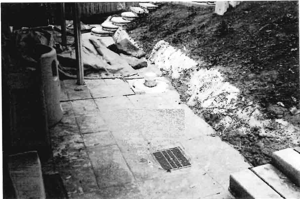
PHOTO 1-4 LOWER PATIO AREA
