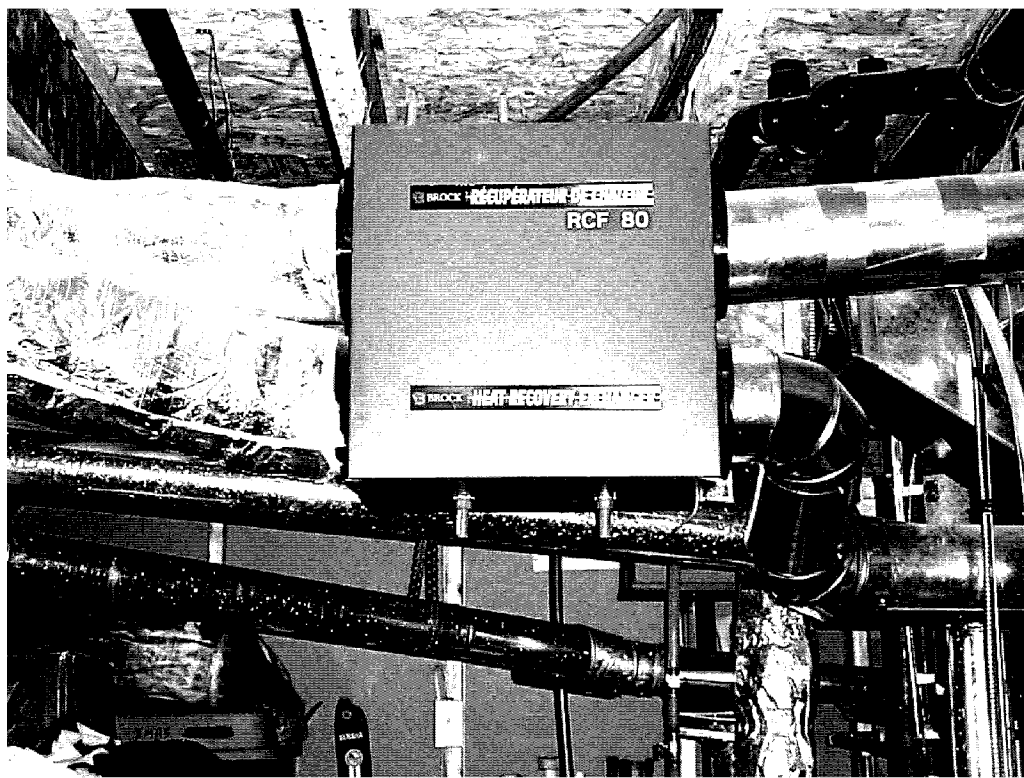
Picture 3 (Passive HRV ventilation system):
