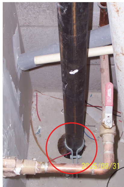
Figure 14: Missing seal around sprinkler riser in garbage room allows unwanted floor-to-floor air movement.
