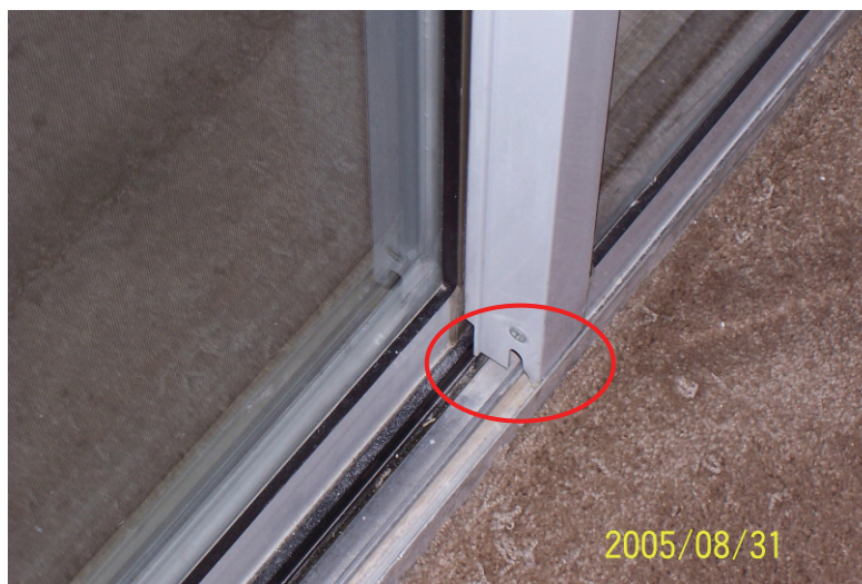
Figure 12: Poor seal along the bottom (and top) of the sliding doors.
