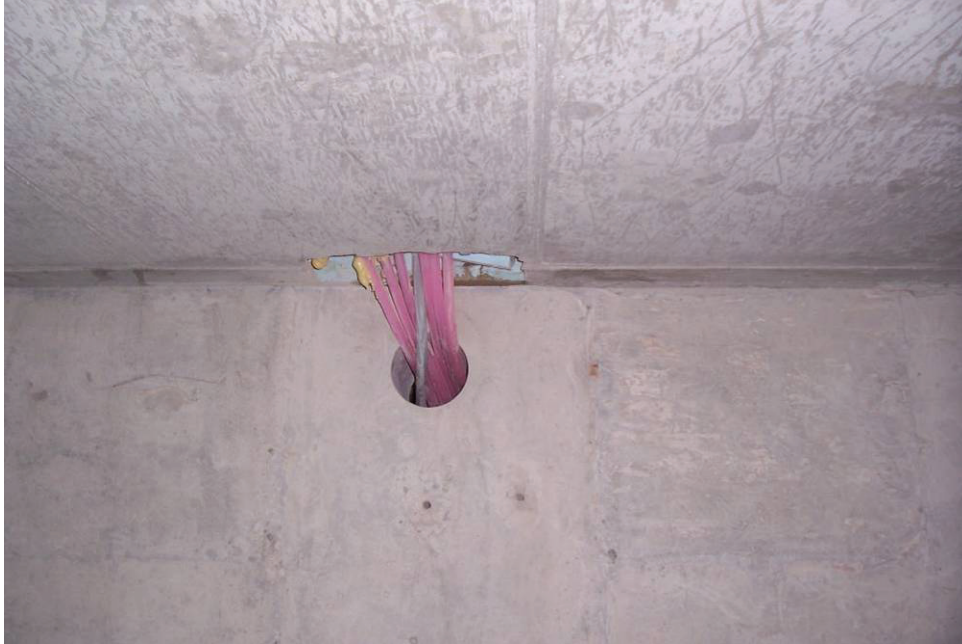
Figure 31: Unsealed opening for electrical cables.
