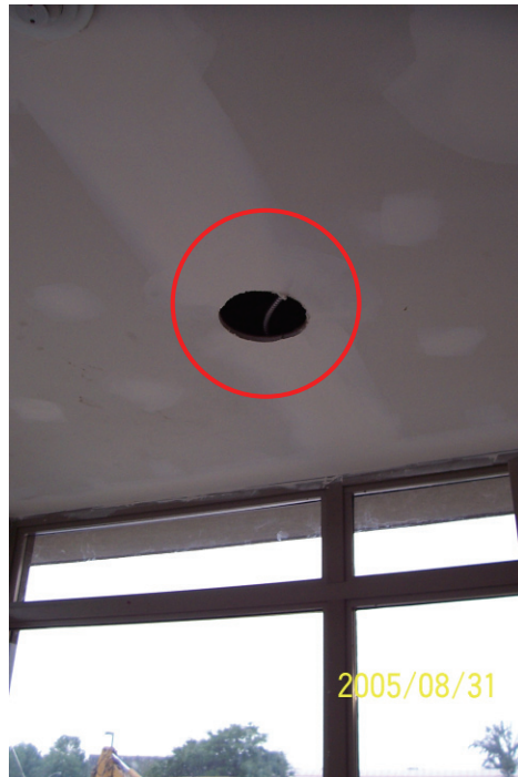
Figure 13: Pot light in the vestibule provides pathway to outside.
