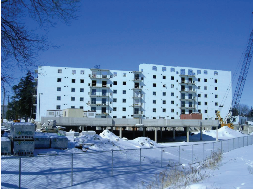
Figure 1: ICF walls being constructed at Cedar Creek apartments.
