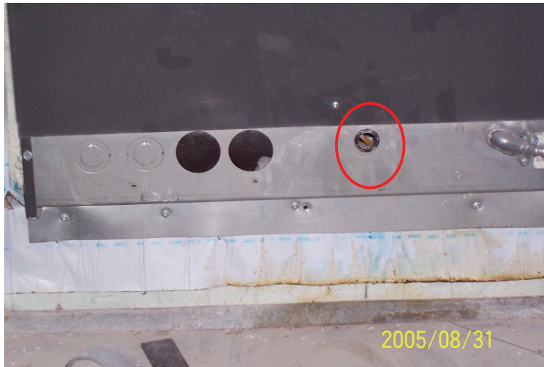
Figure 10: Uncovered knock-out in the condenser cabinet.
