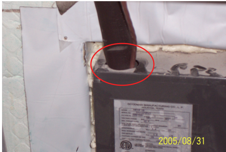
Figure 11: Unsealed opening for condenser refrigerant line.
