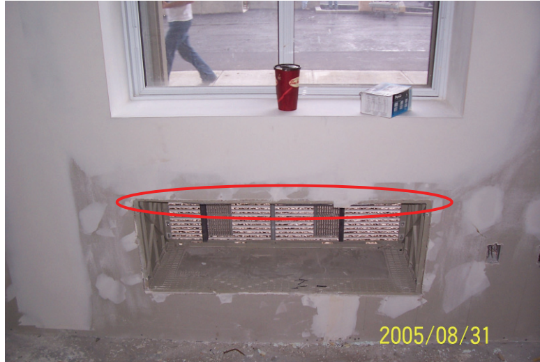
Figure 15: Unsealed front office AC sleeve.
