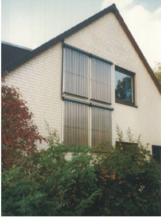
Vertical evacuated collector array as part of a solar combination system
