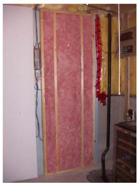
Photo 4.8: No Poly Wall - No evidence of moisture damage.
