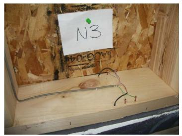
Photo 4.6: Poly Wall North. No evidence of condensation or mold growth
