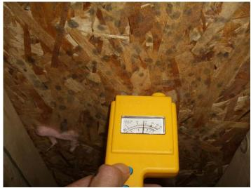
Photo 4.4: No Poly Wall North. Close-up of sheathing showing mold growth.
