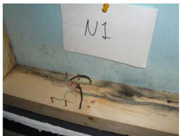
Photo 4.2: XPS Wall North - Mold growth at outboard side of sill plate
