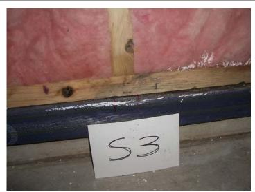
Photo 4.5: Poly Wall South. Mold visible at inboard side of bottom plate, also some visible condensation on the polyethylene
