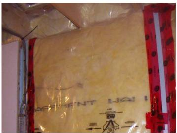
Photo 4.9: Roll Blanket Wall - Discoloration of upper batt (evidence of moisture).
