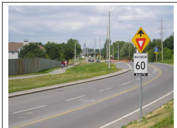
Conventional suburban major collectors are narrow, two-lane roads that do not allow on-street parking.
