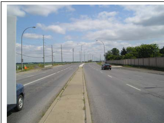
Conventional suburban arterials range from 1-2 lanes with extra lanes around intersections and do not allow on-street parking.
