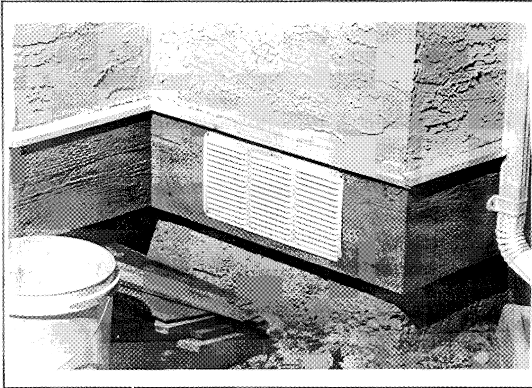
Figure 4: Crawl Space Vent
