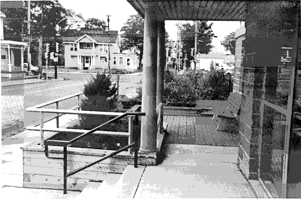
Photo 18 Sheltered entrance lobby at Johnson Manor
