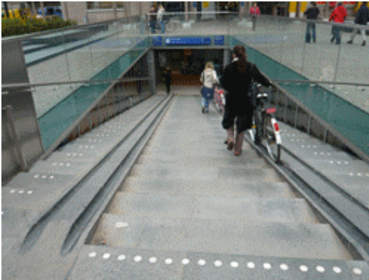
Figure 31 - Access ramp to an underground bicycle station in Amsterdam, Netherlands
