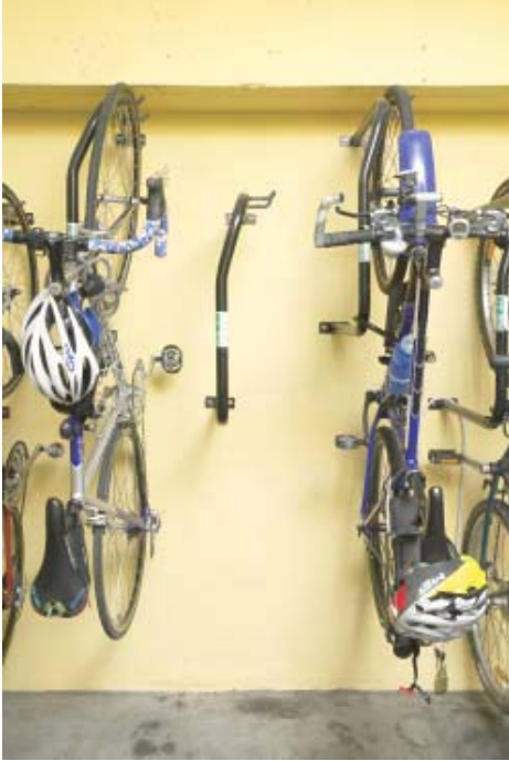
Figure 9 - Wall-mounted bicycle hangers are staggered to prevent handlebar contact between neighbouring bicycles
