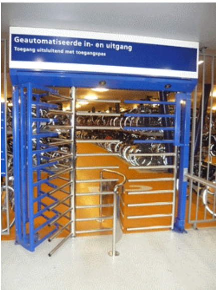
Figure 32 - Swipe card operated access gate at a bicycle station in Amsterdam, Netherlands
