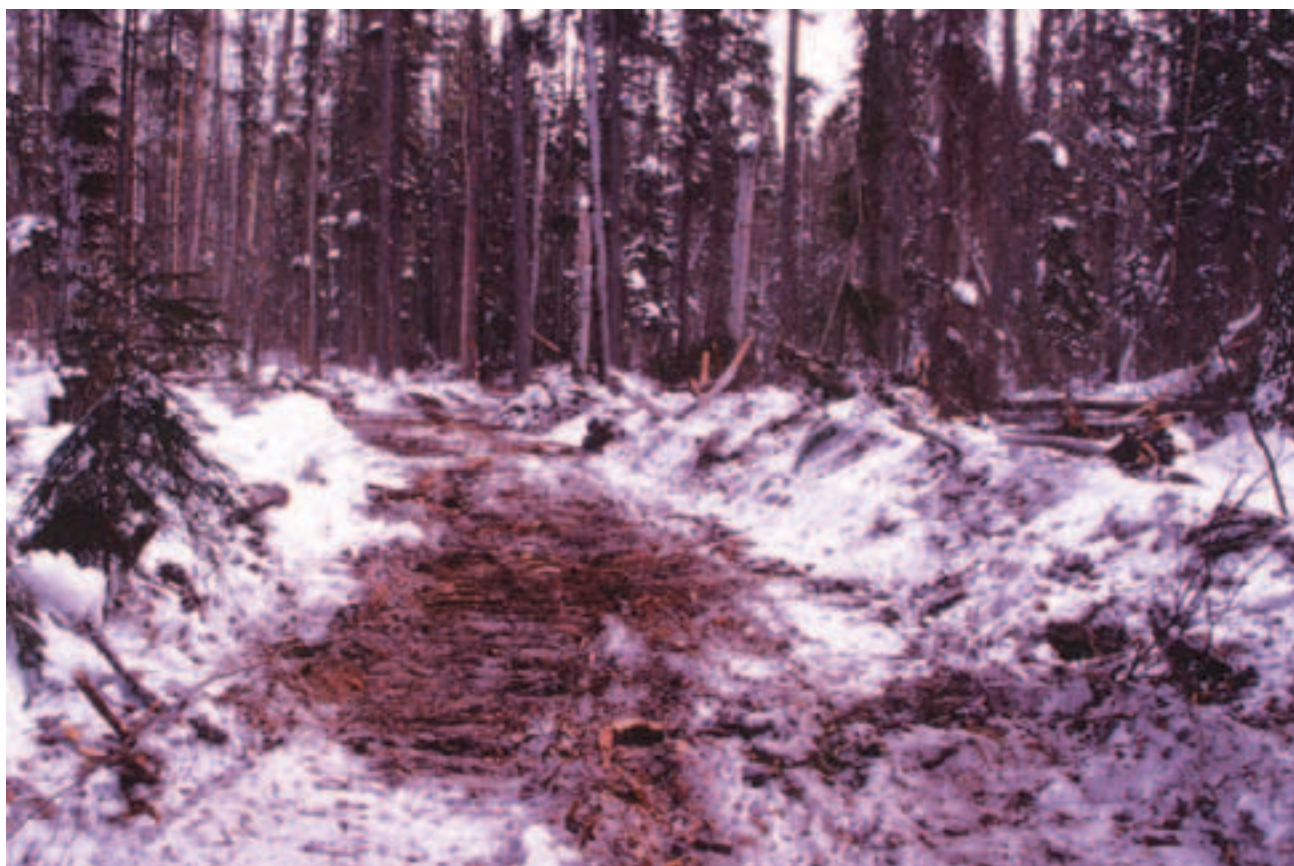
FIGURE 31. On this seismic line, brush is piled in windrows, but standing trees in the piles need to be cut down. More snow or ice is required to protect the ground surface.
