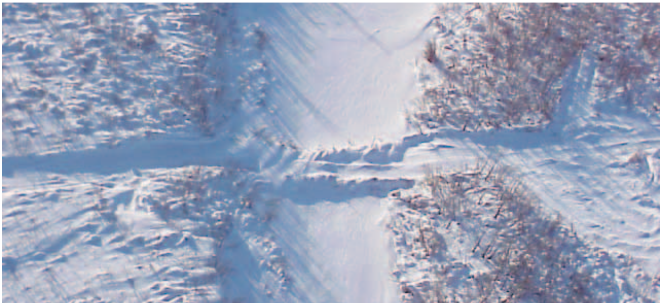
FIGURE 11. A snow fill could have been used at this stream crossing to reduce the bank height and potential for erosion under ice-free conditions.
