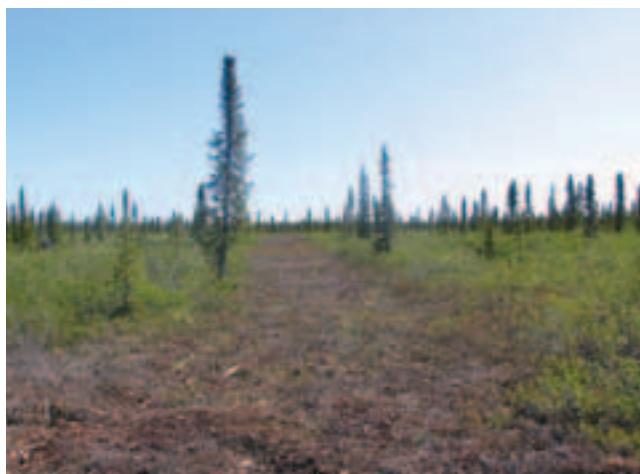
FIGURE 30. (LEFT) A one-year-old seismic line where mulching and scattering was used to dispose of brush. (RIGHT) A seismic line that has been cut with a mulcher in forested terrain. Photo courtesy of Explor.
