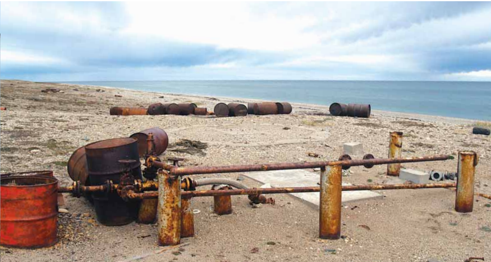
Debris, including barrels and metal piping, litter the PIN-B (Clifton Point) site before remediation.
