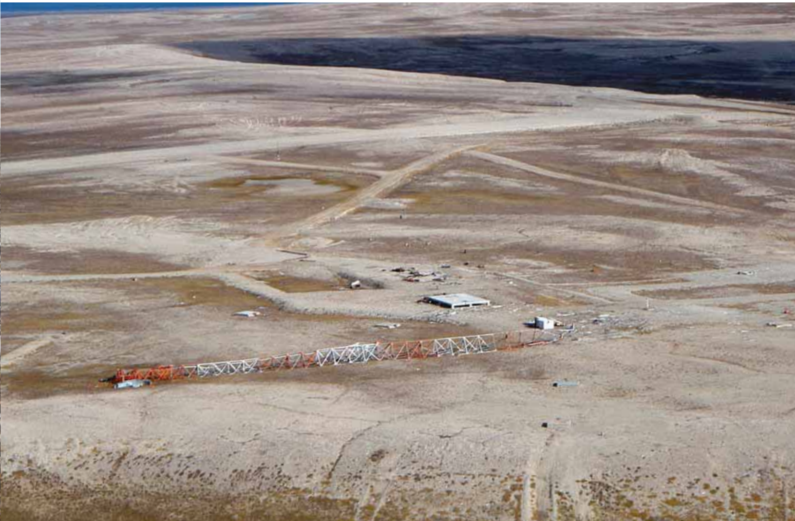
A toppled antennae at the CAM-C (Matheson Point) site.
