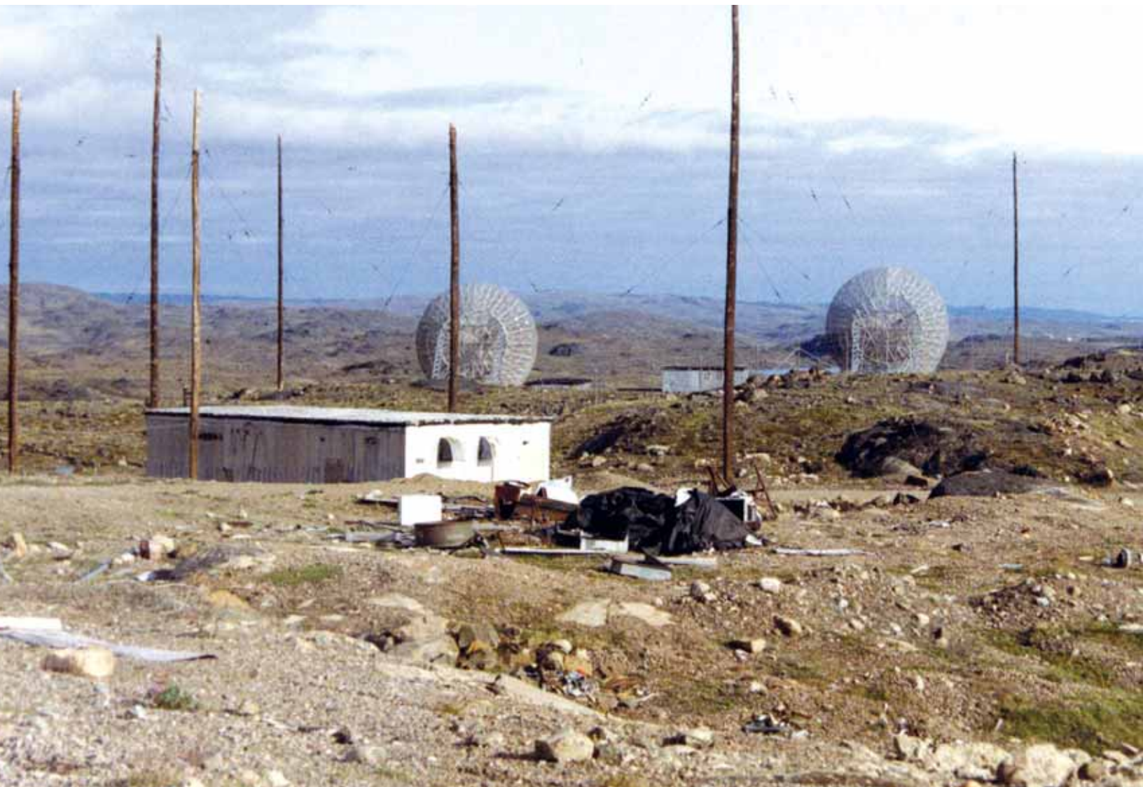
Debris at the Iqaluit Upper Base site prior to remediation.
