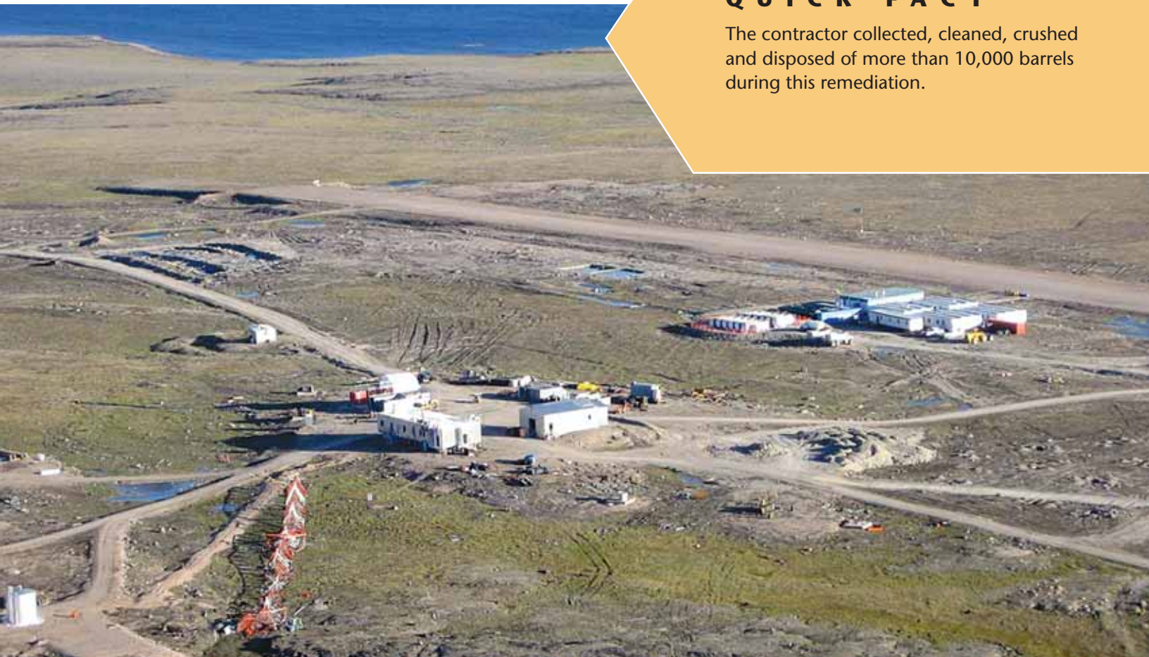
Aerial view of site prior to remediation. These buildings have all been removed.
