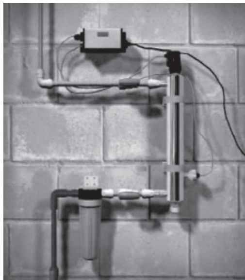
Fig 5.8 A typical UV disinfection system
