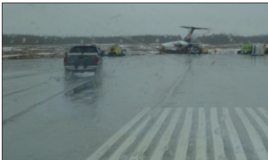
Photo 2. Water visible on Runway 06 (photo taken a few hours after occurrence)
