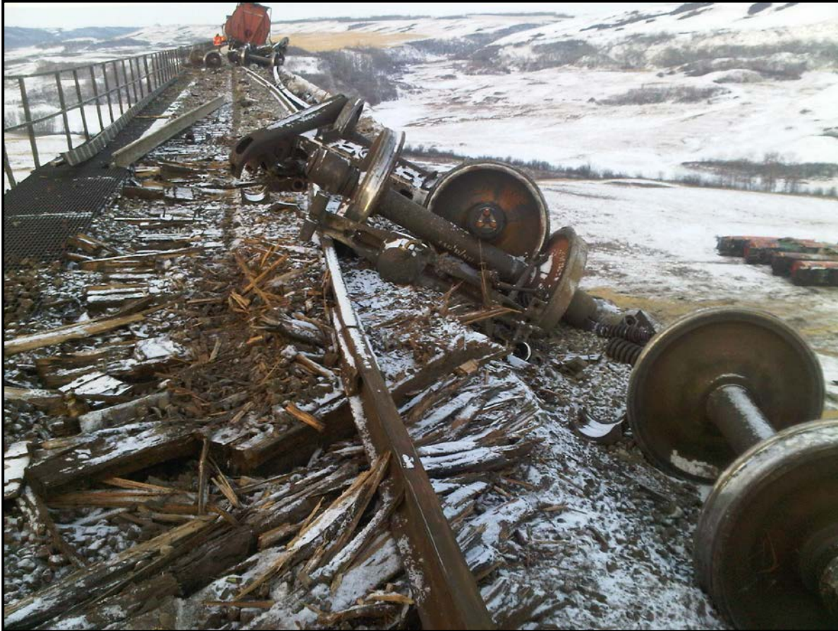
Photo 3. East end of bridge
