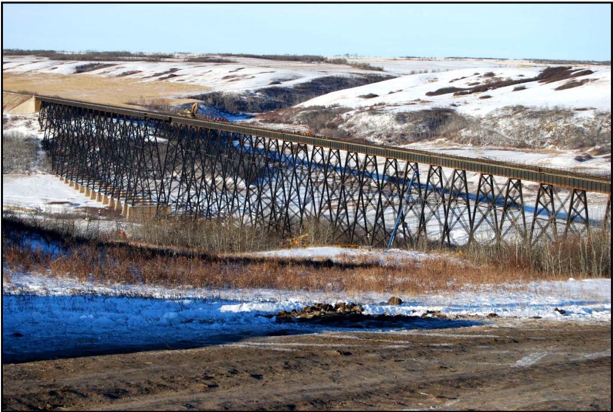
Photo 5. Fabyan Bridge (looking west)
