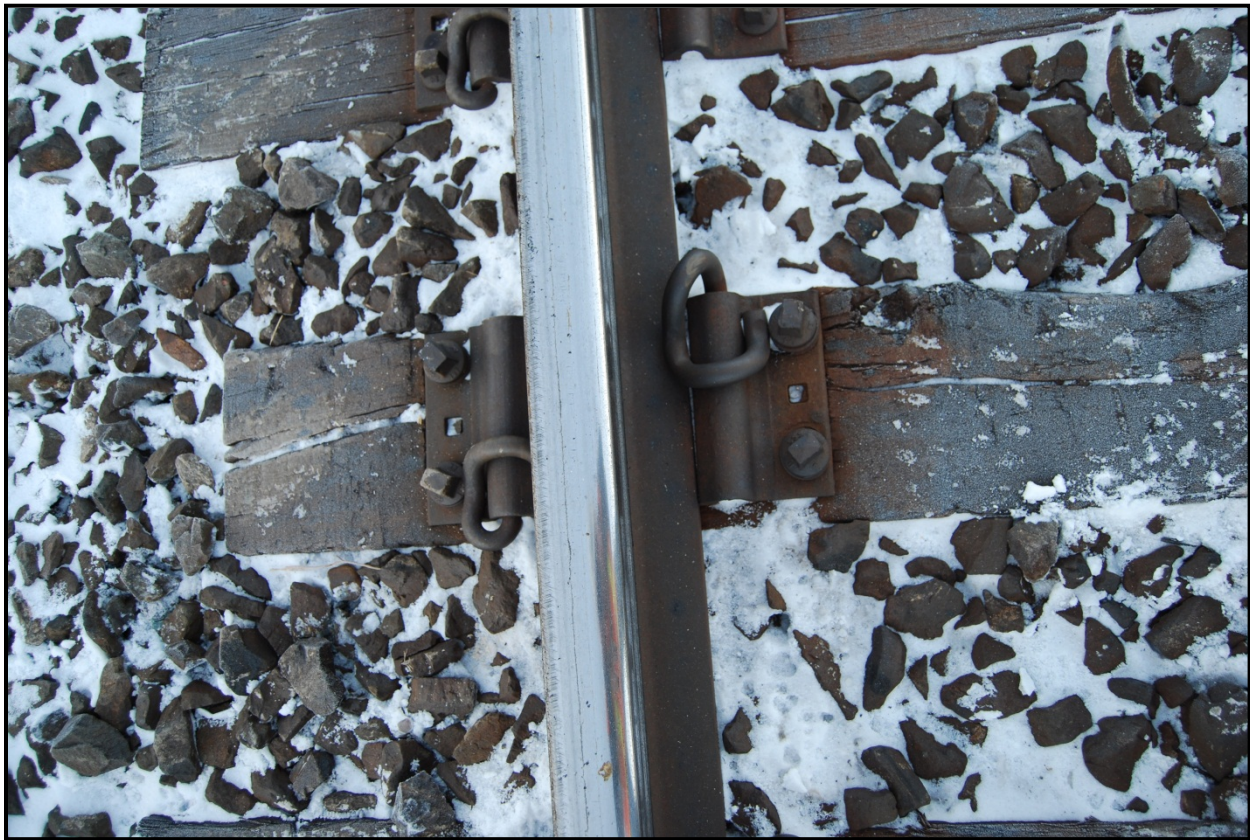
Photo 4. Rolled plate fastener system
