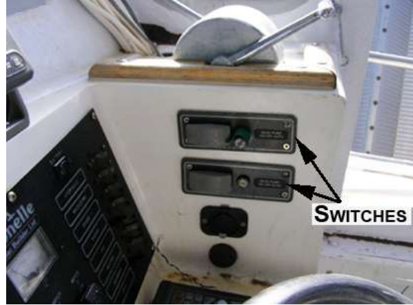
Photo 7. The 2 switches for the electrical pumps in the console area
