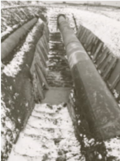
Exposing a pipeline for an integrity inspection
