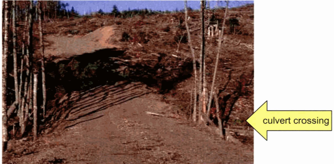
Figure 11: Typical forestry road and culvert crossing in Nova Scotia.
