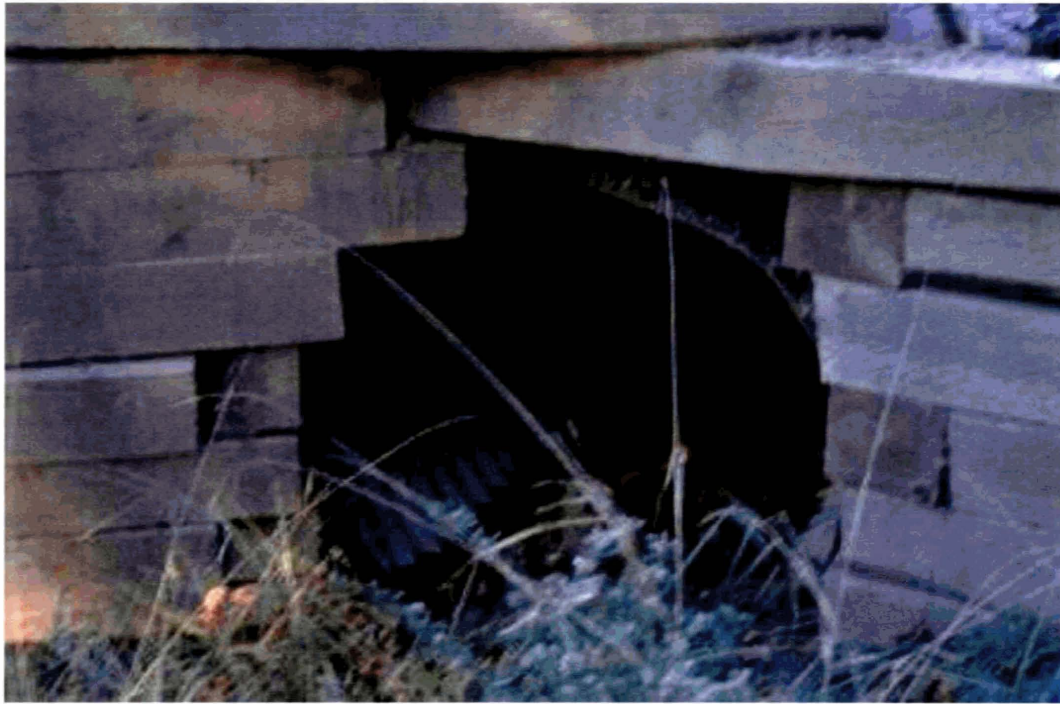
Figure 17: Innovative ideas for stabilization in difficult soils.
