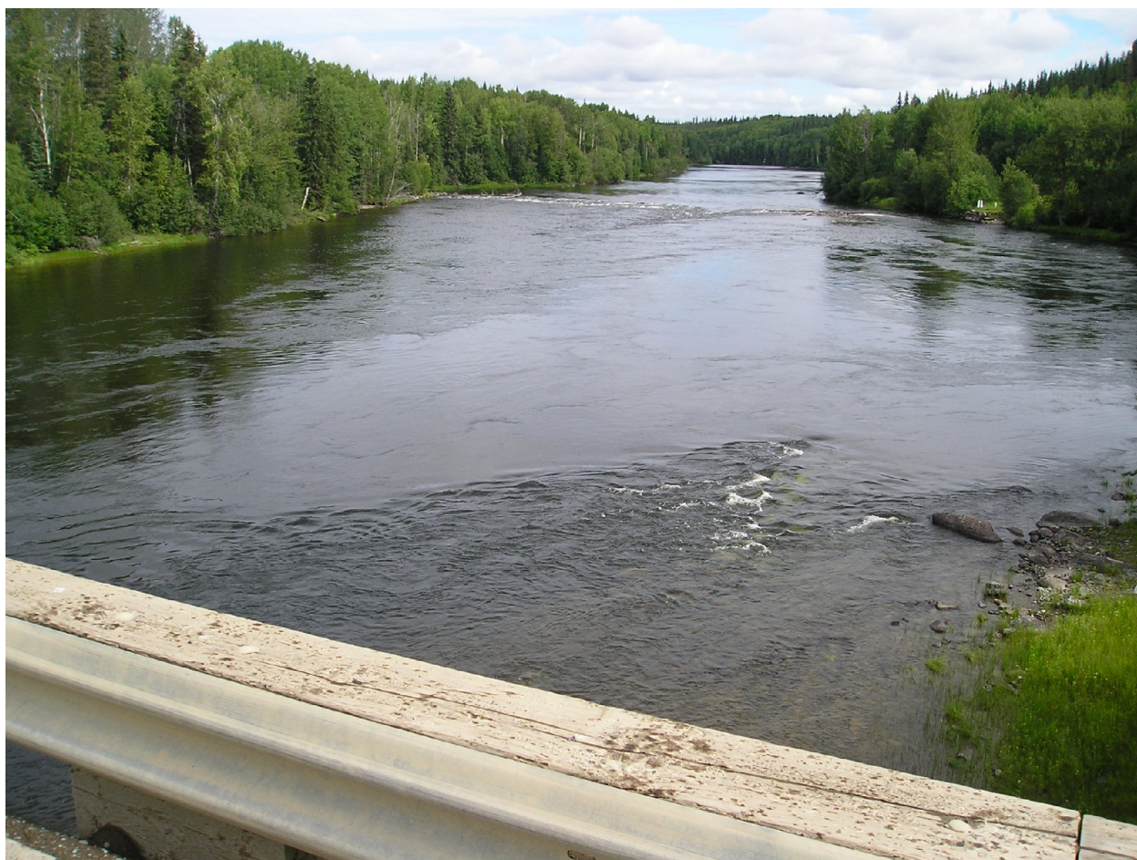
Figure 25. Tachie River on the upstream side of the Tanzuil Road bridge. Picture taken near the left bank on 21 July 2004.
