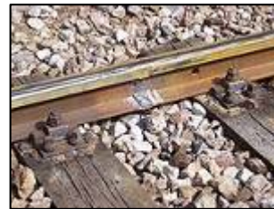
Continuously welded track
