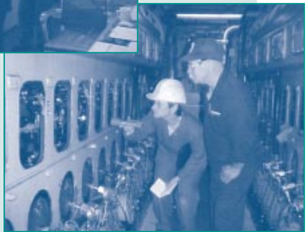
Leah Quiring observing tests on a main electrical switch board (top) and inspecting a fuel injection system (bottom).
