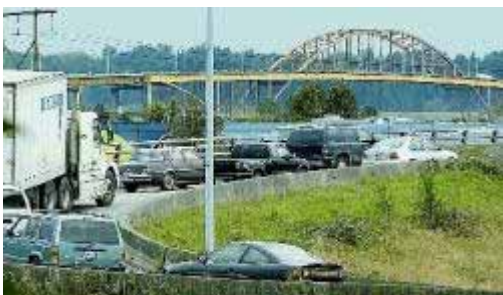
Short queue jump HOV lanes can be a cost effective congestion management approach at common traffic choke points, such as this bridge approach in Vancouver.
