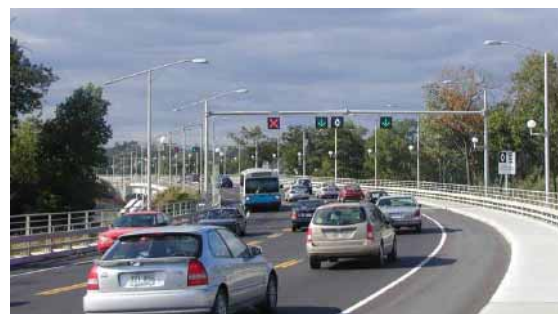
Counter-Flow HOV Lane, Ottawa
